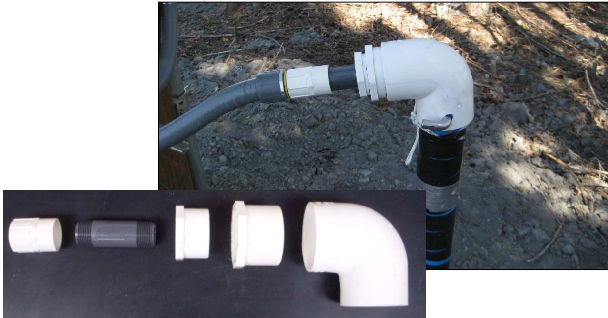
Figure A-18. Guide casing to flexible conduit adapter in place on TH09-1511 casing. Inset illustrates the various PVC fittings that comprise the adapter. (Photographs by M. Darrow, May 2010)
