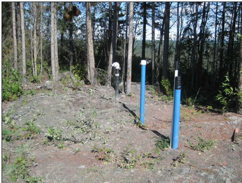
Figure A-23. Final configuration of the Rich113 site in August 2011. The post that supported the ADAS was cut off at the ground surface. Only the guide casings remain for manual inclinometer probe readings. (Photograph by M. Darrow)
