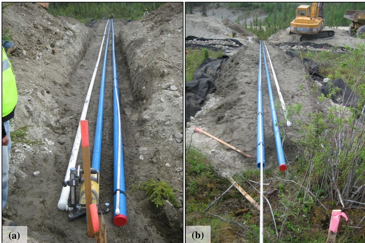
Figure C-2. Casings prior to backfill at the instrumented cross section, looking (a) upslope and (b) downslope. (Photographs by M. Darrow, June 2012)
