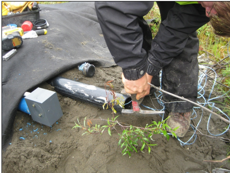
Figure C-15. Tapping ABS end cap adapter into the sand bedding to be flush with inner casing. (Photograph courtesy of J. Zottola, July 2012)
