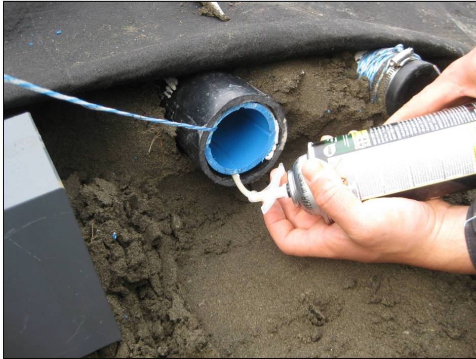
Figure C-16. Filling annulus space with expanding foam to seal outer ABS end cap adapter in place. (Photograph courtesy of J. Zottola, July 2012)
