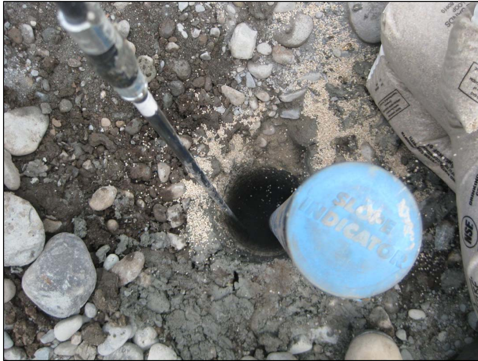
Figure B-1. Tamping dry sand backfill around the guide casing. (Photograph by M. Darrow, June 2010)
