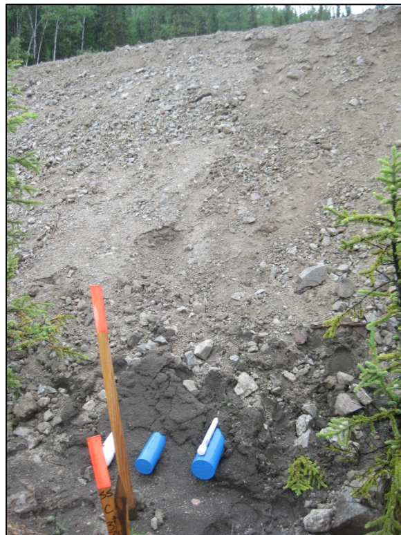
Figure C-4. Downhill toe of embankment with thermal berm and exposed casing ends. (Photograph by M. Darrow, July 2012)
