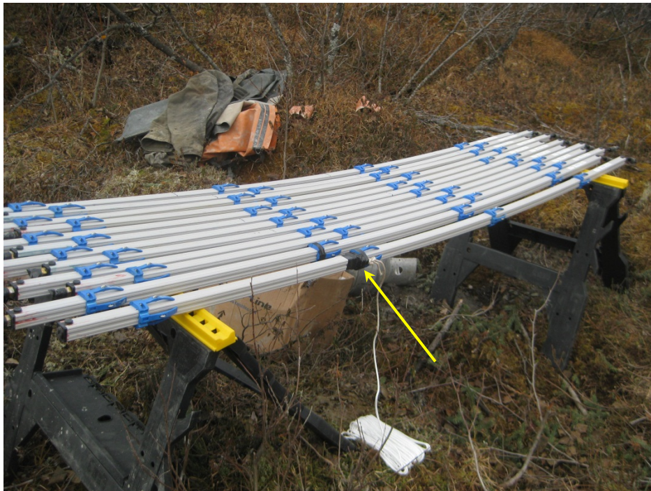
Figure D-3. INC500 modules, staged and ready for installation. A safety line was attached to the lowest module (indicated by the yellow arrow). (Photograph by M. Darrow, Sept. 2012)
