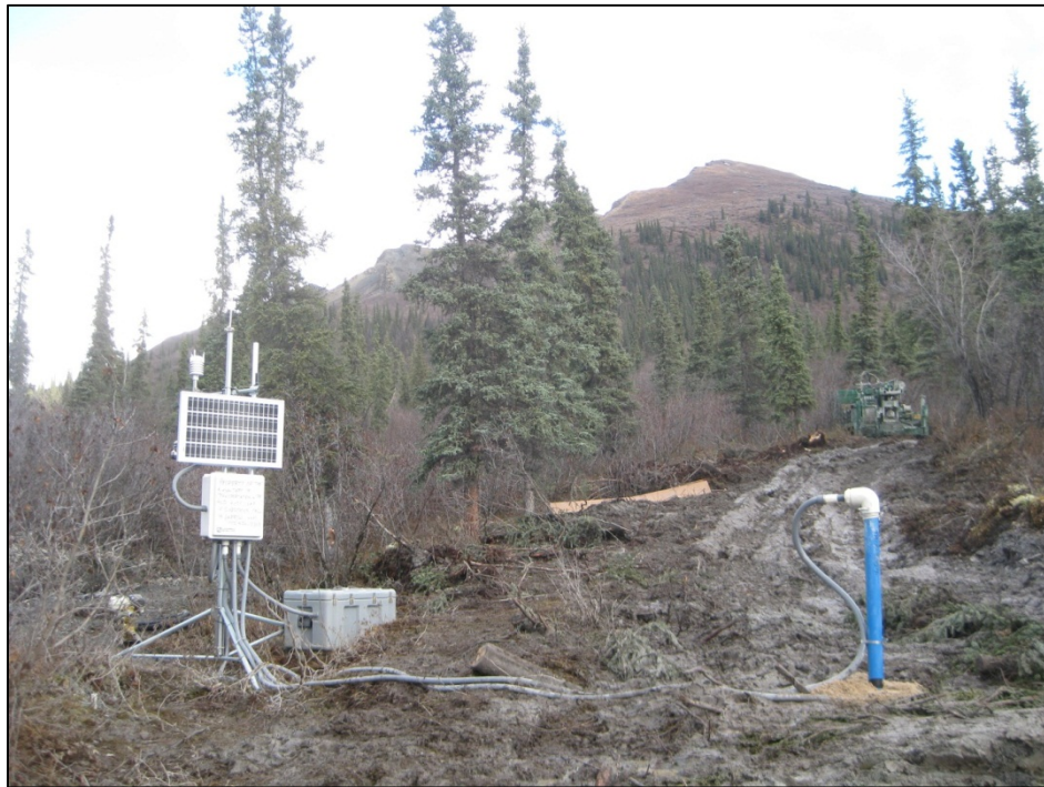
Figure D-7. Completed ADAS location and casing installation of TH12-9004. (Photograph by M. Darrow, Sept. 2012)
