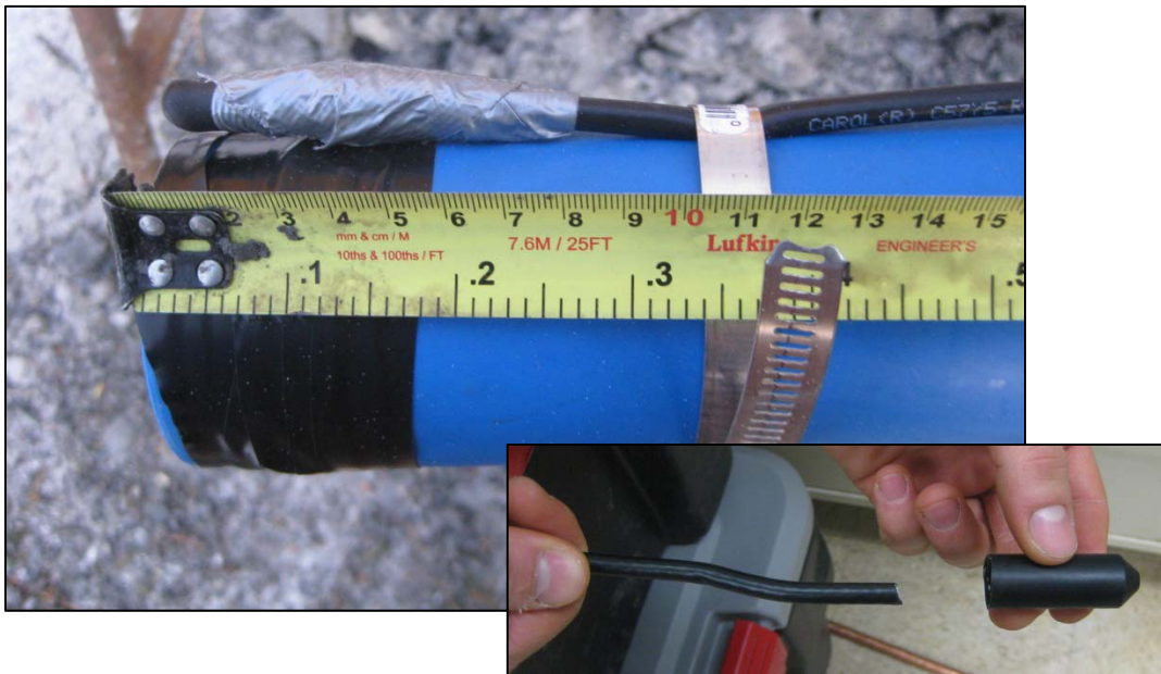
Figure A-2. Configuration of coaxial (TDR) cable at the bottom of the guide casing prior to installation. Inset illustrates sealing the cable end with an adhesive cap. (Photographs by M. Darrow, Nov. 2009)
