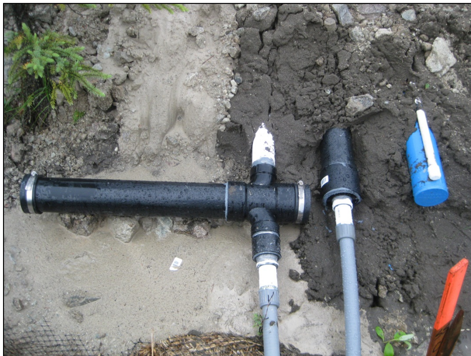
Figure C-12. PVC casing to flexible conduit adapter for SAA installation. (Photograph by M. Darrow, July 2012)
