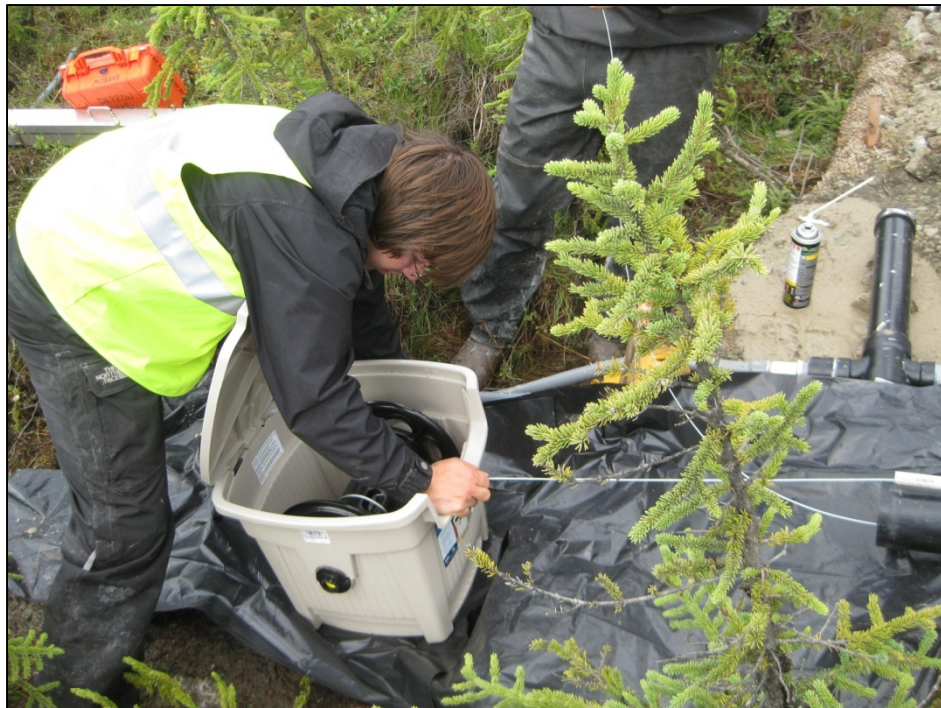
Figure C-21. Winding up excess wire rope from within casing assembly. (Photograph by M. Darrow, July 2012)
