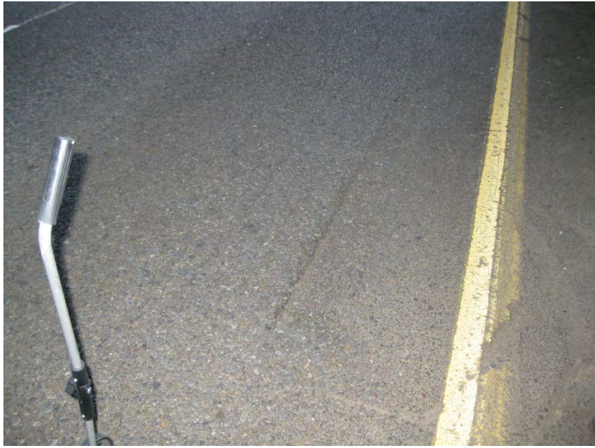
Photo 1164 (Station 37+25, looking east)
