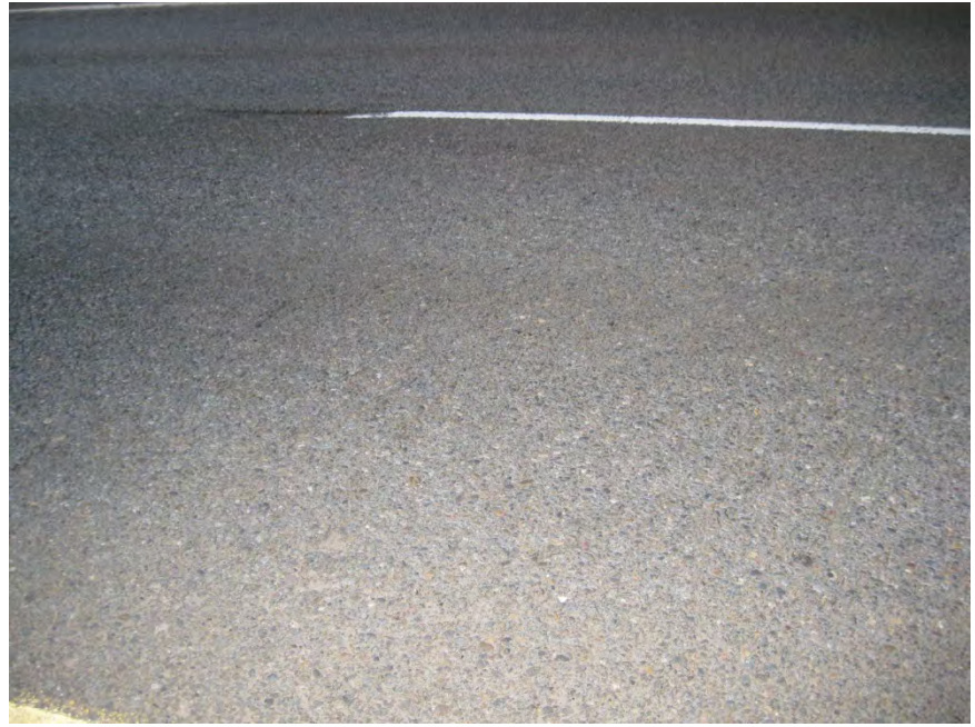
Photo 1165 (Station 38+00, looking east)
