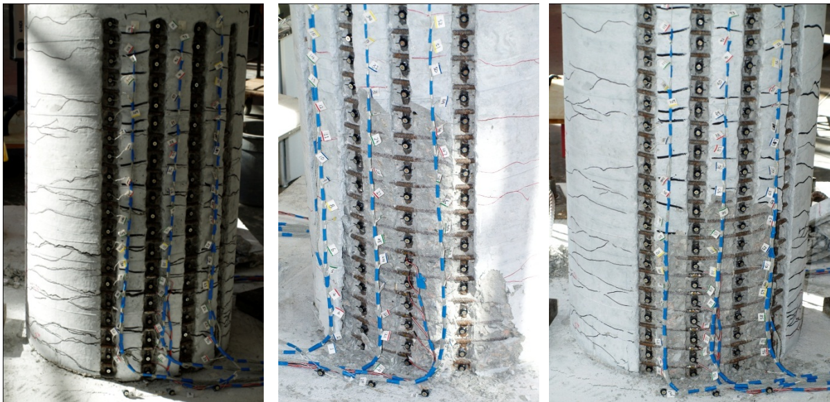
Figure 2-108. Test 11 – (Left and Middle) North and South Sides of Specimen during ( \mu_{10}^{3.86 \text{ sec}} = 8.28'' ) and (Right) North Side of the Specimen during ( \mu_{-6.1}^{4.42 \text{ sec}} = -5.08'' )
