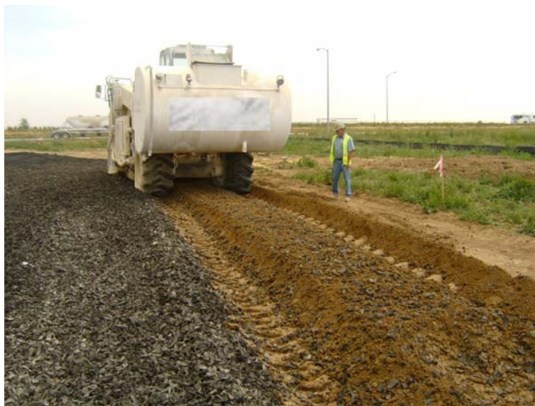
Figure 9. Rotary tiller typically used in lime/fly ash stabilization employed during field construction of an tire chip-ESR stabilized subgrade layer
