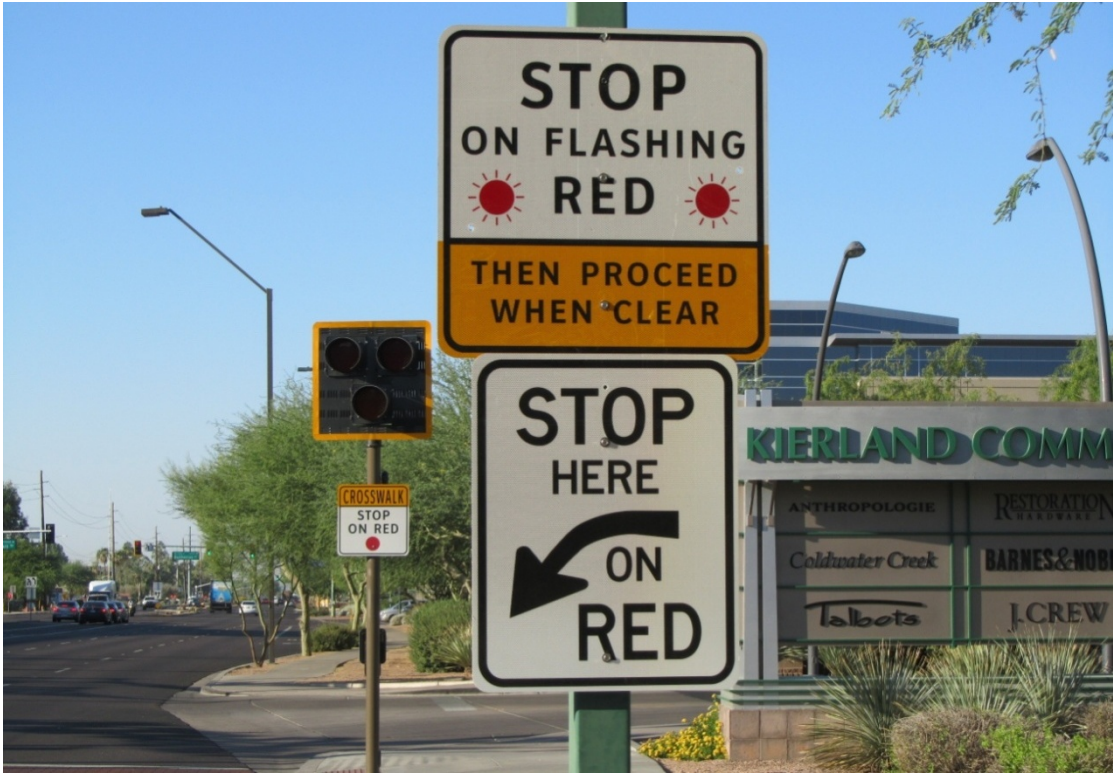
Figure 5-1: An example of a sign to explain the flashing red indication at a PHB.
