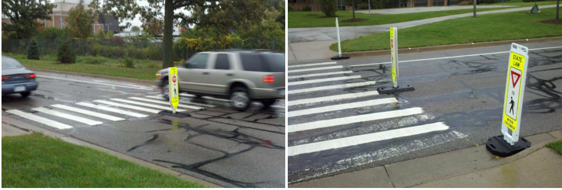
Figure 3-1: The left frame shows the installation with one sign and the right frame shows the Gateway installation with three signs.
