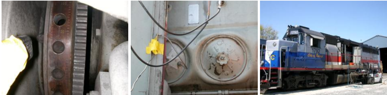
Figure 3-12. Installation of Sensors on a GP40 Locomotive Prime Mover Engine (a) engine RPM sensor; (b) manifold absolute pressure (MAP) sensor; (c) side-view of locomotive
