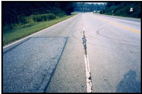
Figure 5-11: Raveled longitudinal joint (Brown, 2006).
