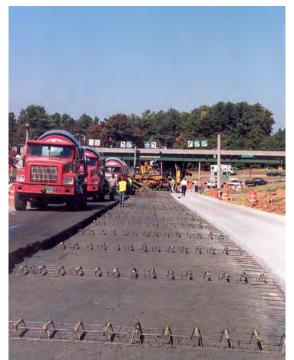
Figure 5-2: Dowels can be placed within acceptable tolerances, field measurement every day is critical.
