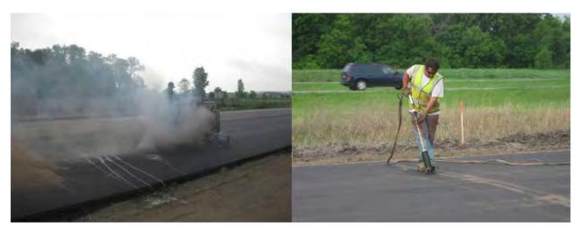
Figure 5-15: Sawing joints in the AC layer which correspond to the joints in the underlying PCC layer (left) and sealing the newly sawn joints (from Rao et al 2011).
