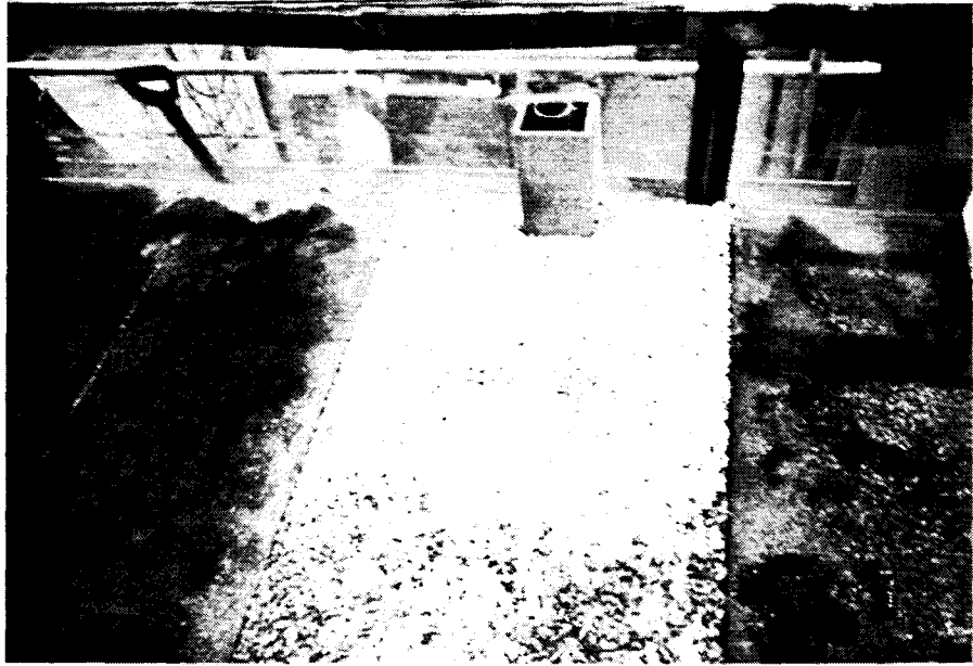
Figure 17. View of typical setup for the vertical wall abutment in the observation area.
