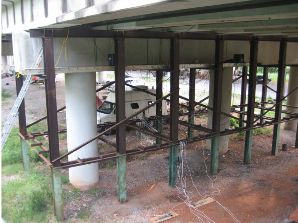
Figure F-2: View of false supports under Bent 11
