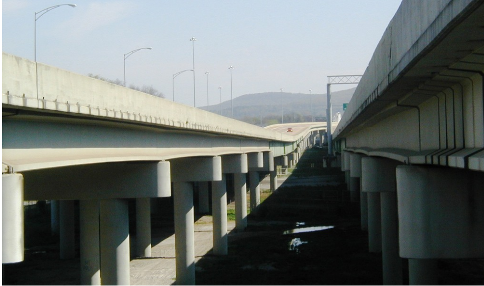
Figure 1-1: Elevated spans of I-565 bridge in Huntsville, Alabama
