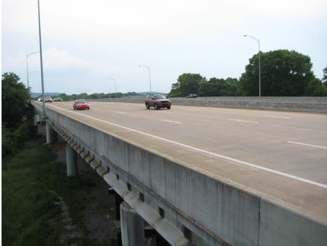
Figure F-1: View of I-565 bridge structure
