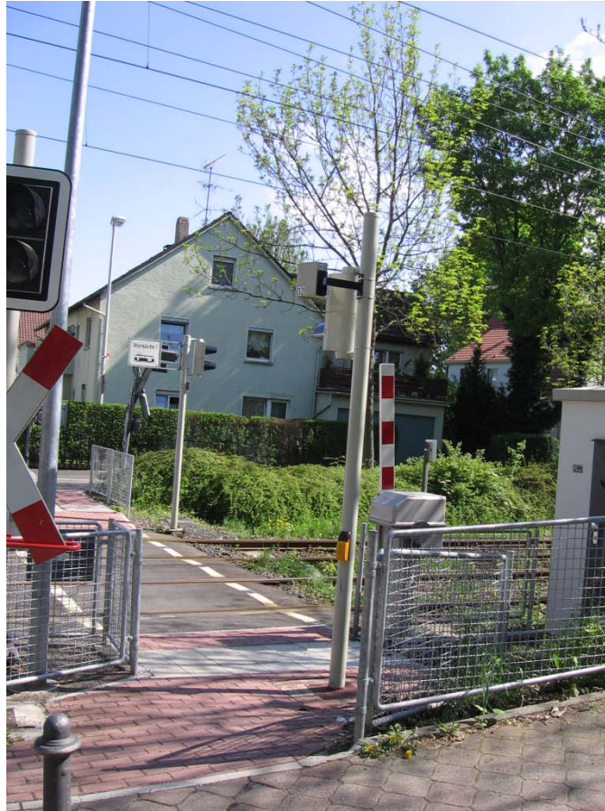
Figure 6. Pedestrian Crossing with Barrier and Acoustic Warning for the Visually Impaired.
