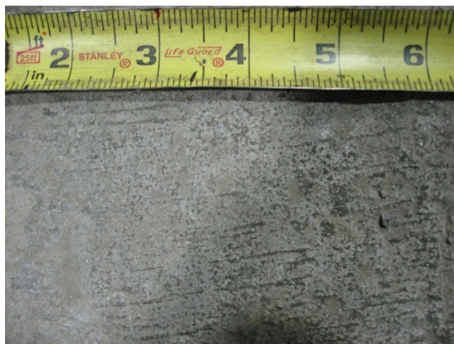
Figure 2.8. Concrete surface finish
