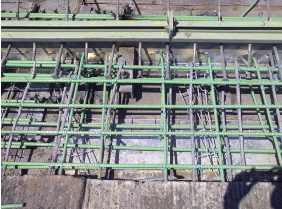
Figure 2-8: A dam with all new reinforcement installed
