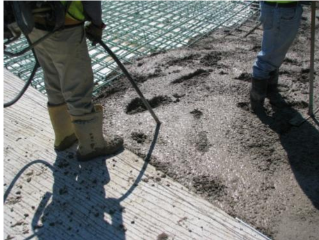
Figure 2-2: Vibrating the approach slab on the opposite end of the deck
