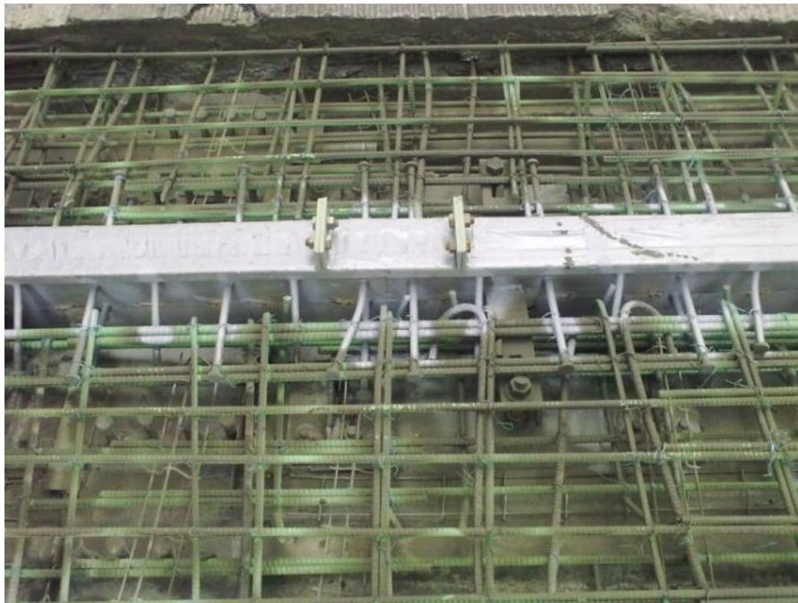
Figure 2-9: Both sides of a dam with new reinforcement installed
