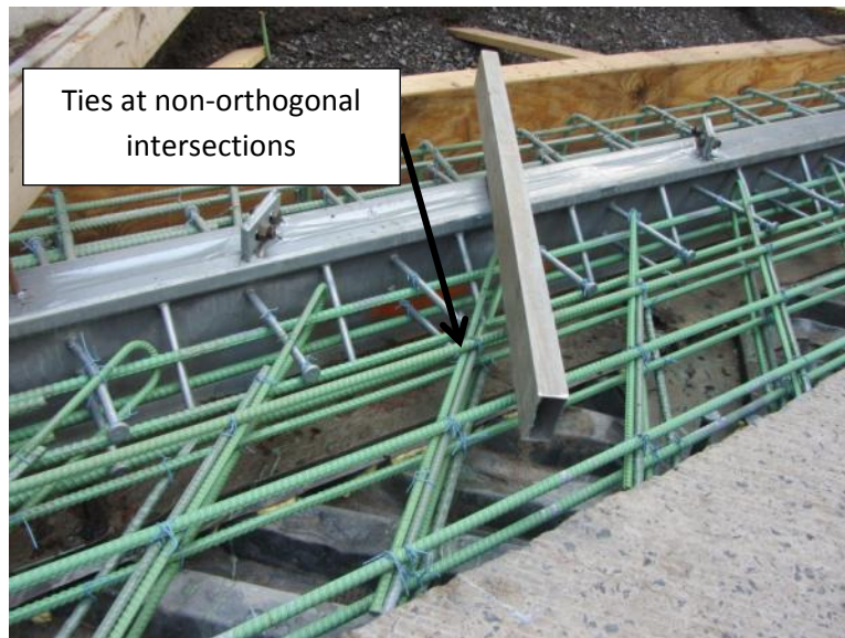
Figure 2-17: Final placement of bridge dam
