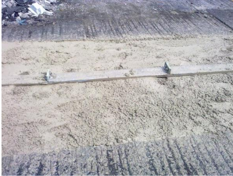
Figure 2-12: The rough finish of the first dam
