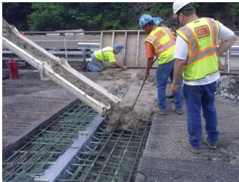
Figure 2-11: First dam's pouring, vibration, and finishing
