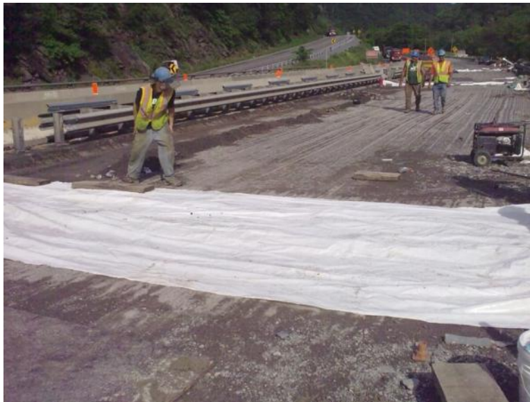
Figure 2-16: Final white plastic sheeting cover
