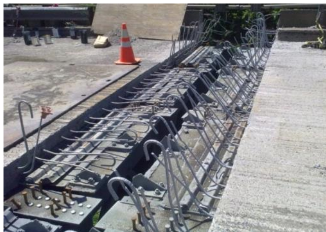
Figure 2-3: Repair area of bridge deck with old dam and concrete removed
