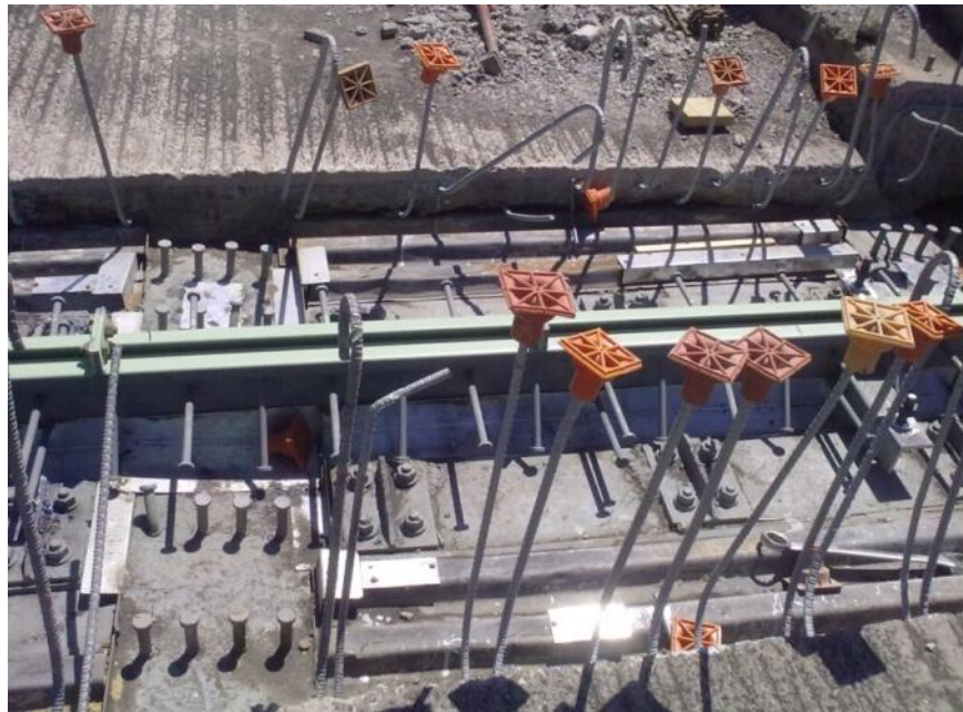
Figure 2-5: New dam hardware after installation
