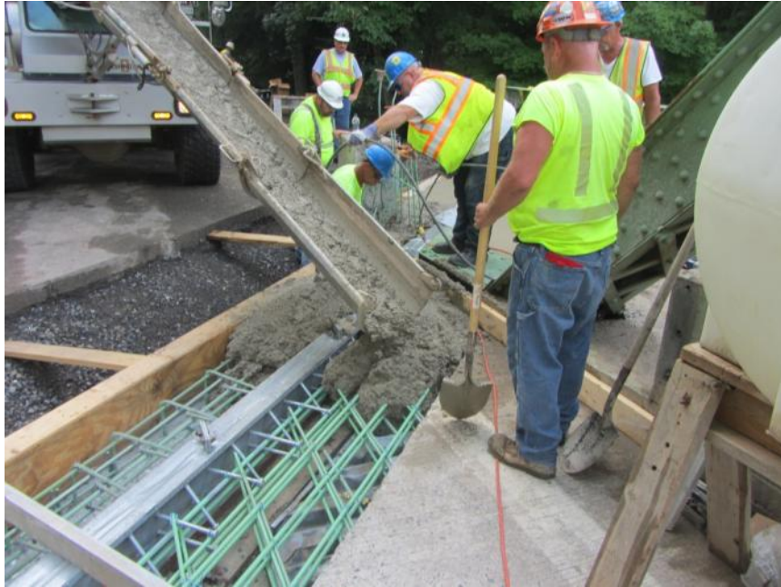
Figure 2-20: Placement of concrete blockout adjacent to bridge dam
