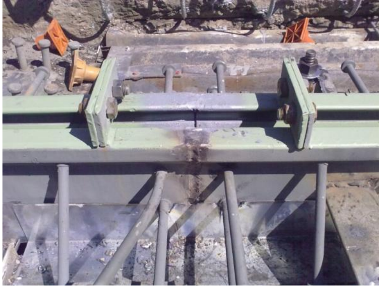
Figure 2-6: Welded dam sections
