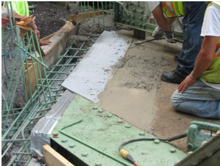
Figure 2-21: Compacting concrete by vibration
