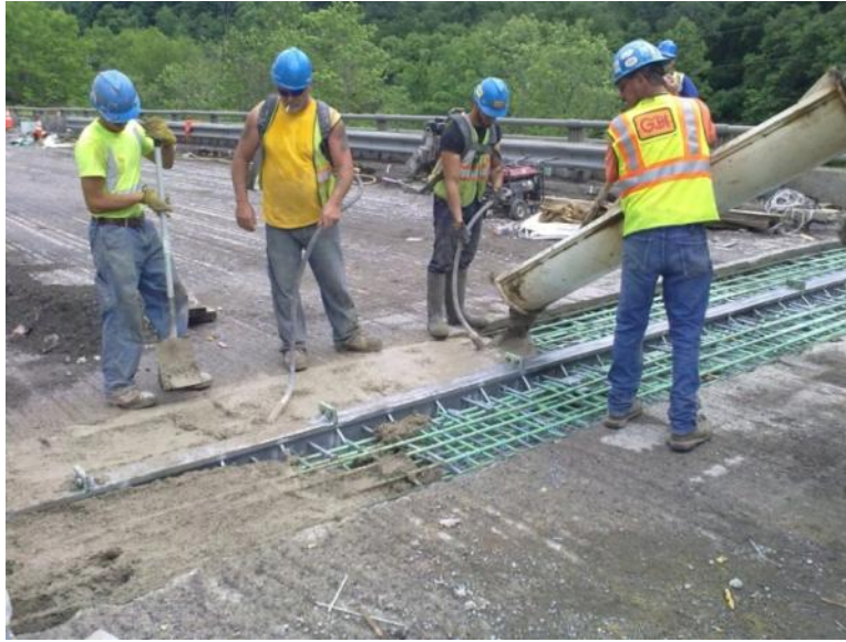
Figure 2-13: Placing and vibrating concrete from the third truck
