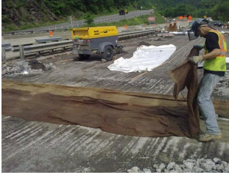
Figure 2-15: Spreading the wet burlap on the finished surface
