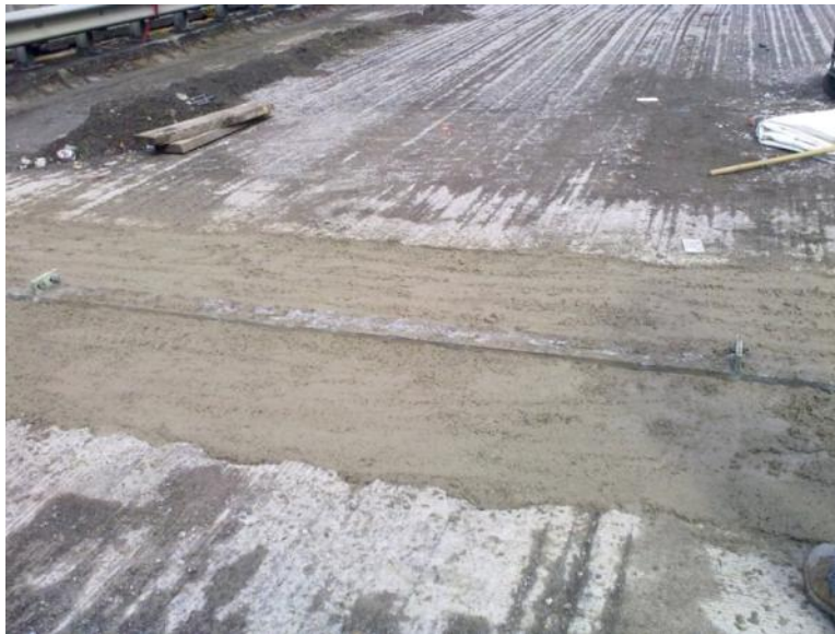
Figure 2-14: The rough finish of the second dam
