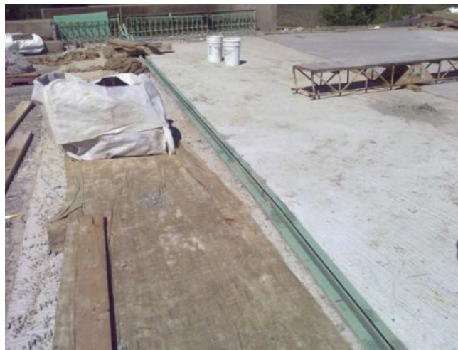
Figure 2-1: A completed bridge deck dam replacement
