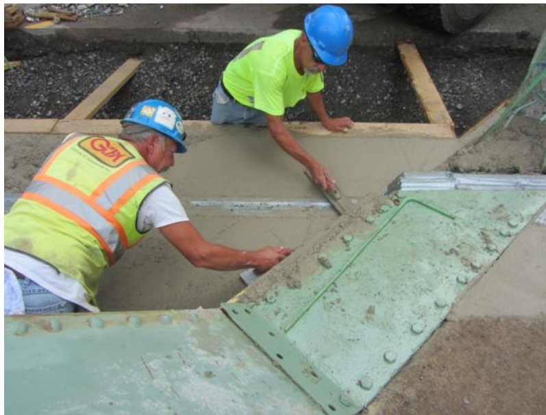
Figure 2-19: Finishing concrete to grade
