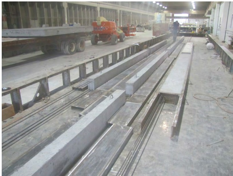
Figure 4.9 – Beams After Form Removal and Before Instrumentation
