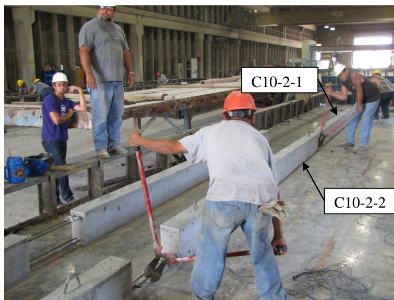
Figure 5.14 – Release of C10-2 Beams
