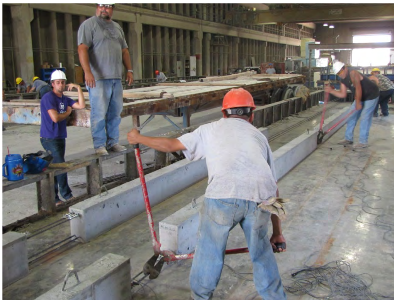
Figure 4.10 – Bolt Cutting Strands at Release
