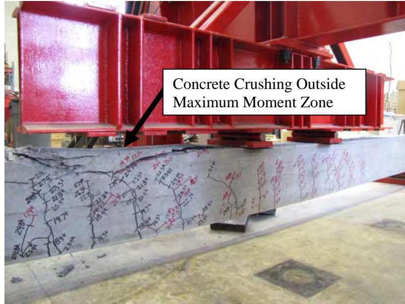
Figure F.15 – S6-2-2_73 at Failure
