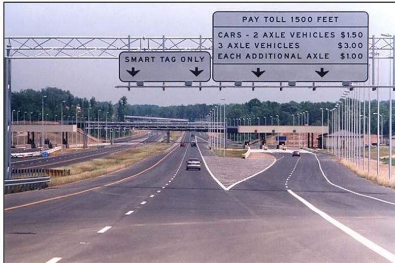
Figure 2-6. A combination facility, which includes open-road tolling and booths
