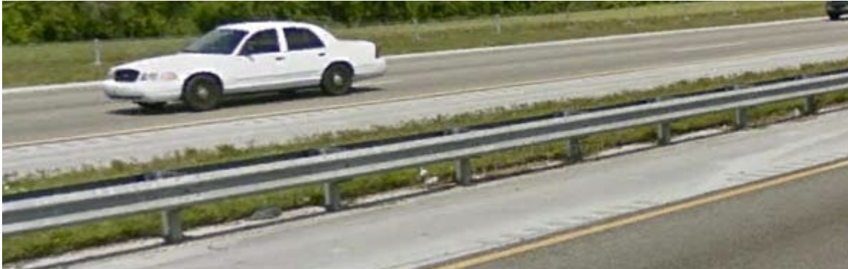
Figure 1-1: G4 (1S) Strong-post W-beam Guardrail without a Rub-rail on Florida Turnpike in Miami-Dade County
