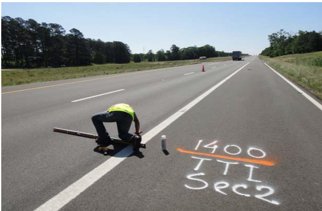
Figure 2 Balanced mix design results from the Atlanta District. Increasing the design asphalt content 0.3% doubled the OT cycles to failure. The modified mix is performing very well after 2 years of service on US 59.
