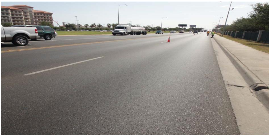
Figure 1 Balanced mix design results for a Type C mix with RAP from the Laredo District. No satisfactory results could be obtained from the PG 70-22 binder so a change was made to the PG 64-22 binder with a reported savings of $5 per ton. US 59 section after 2 year is shown above.
