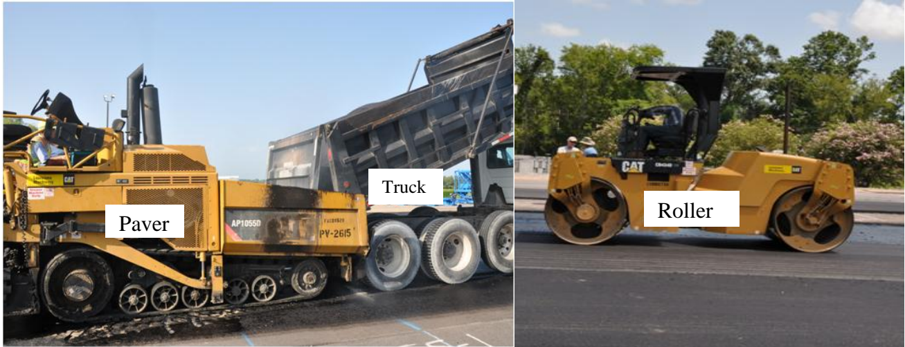
Figure D-3. HMA Placement of the APT Test Sections.
