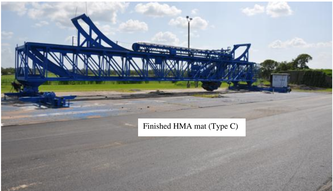
Figure D-4. Finished HMA Mat on the APT Test Sections.
