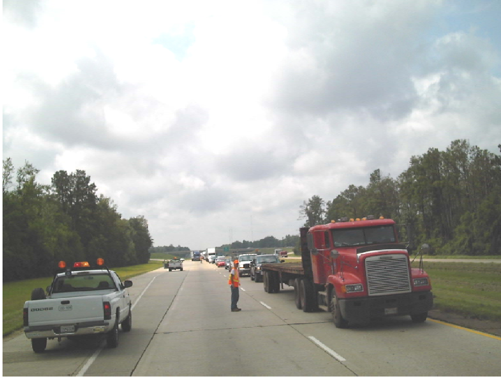
Figure 11 Flaggers near the installation of MIRs
