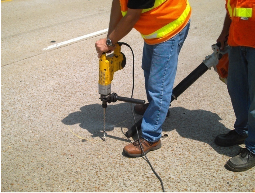
Figure 12 Example of the installation process
