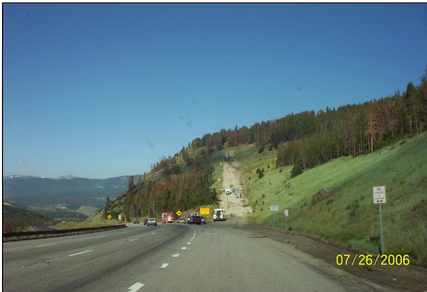
Figure 1.3 Perhaps the most-used runaway ramp in Colorado: the western side of the Eisenhower tunnel on I-70 just east of Silverthorne, showing a maintenance crew after an event. This ramp has over 20 reported events per year, with 106 reported 2001-2004.
