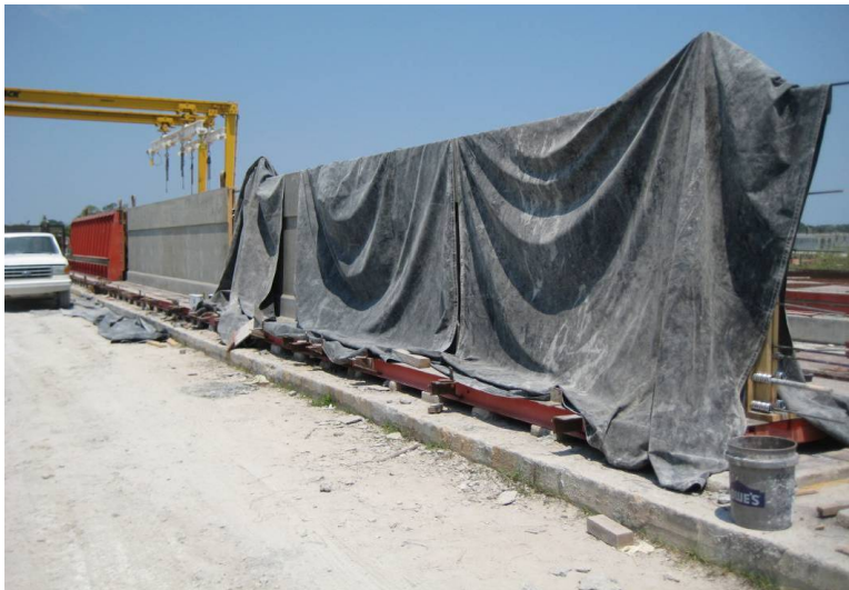
Figure 10.5. Tarp covers applied to each segment during curing
