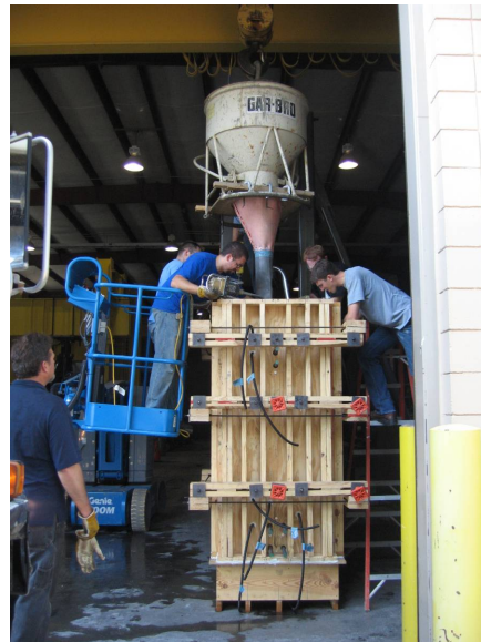
Figure 10.18. Placement of concrete in north end block formwork
