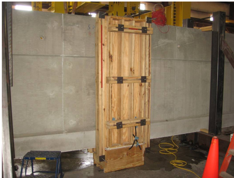
Figure 10.10. Closure strip formwork
