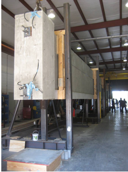
Figure 10.29. Lifting the test girder into testing position, prior to end block fabrication
