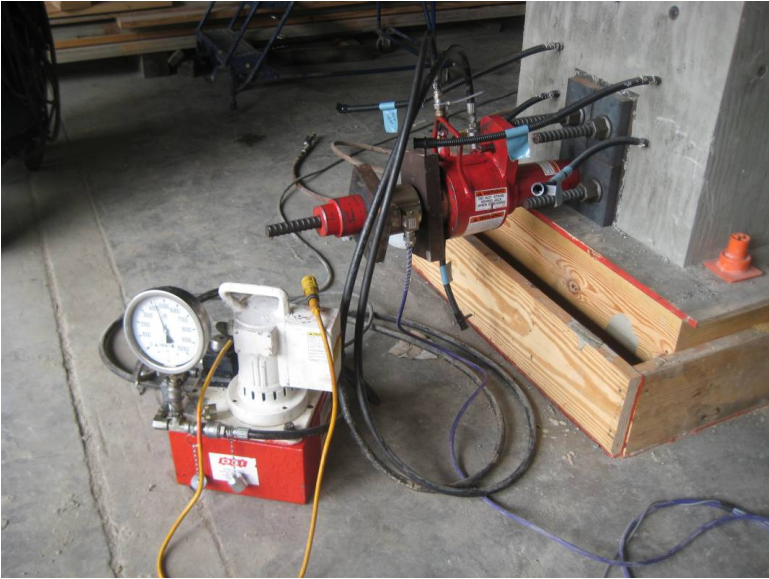
Figure 10.26. Post-tensioning jack and pressure gage
