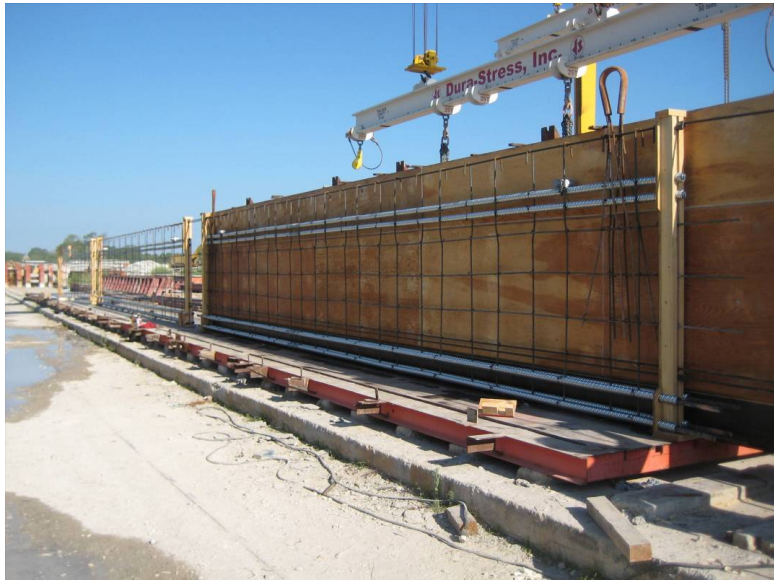
Figure 10.2. Precast segments formwork aligned on single pretensioning bed at Dura-Stress
