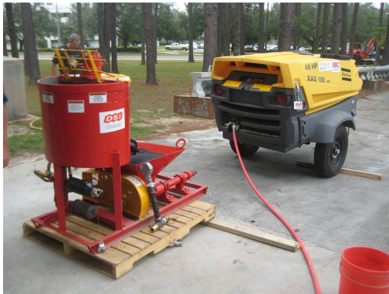
Figure 10.28. Grout mixer and high capacity air compressor
