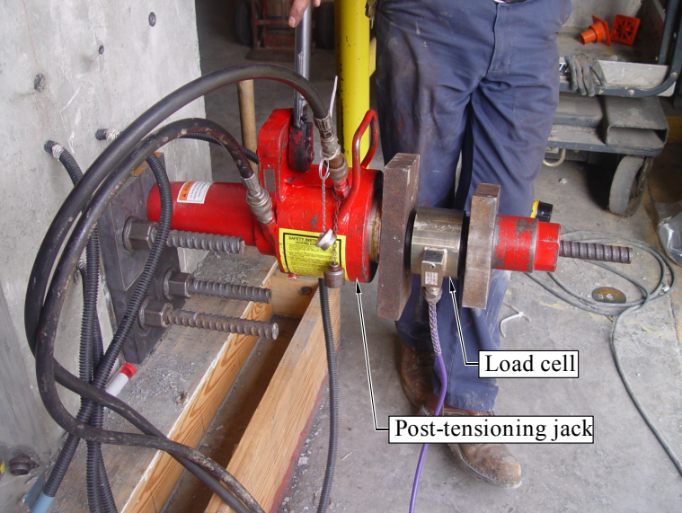
Figure 10.25. Post-tensioning jack setup
