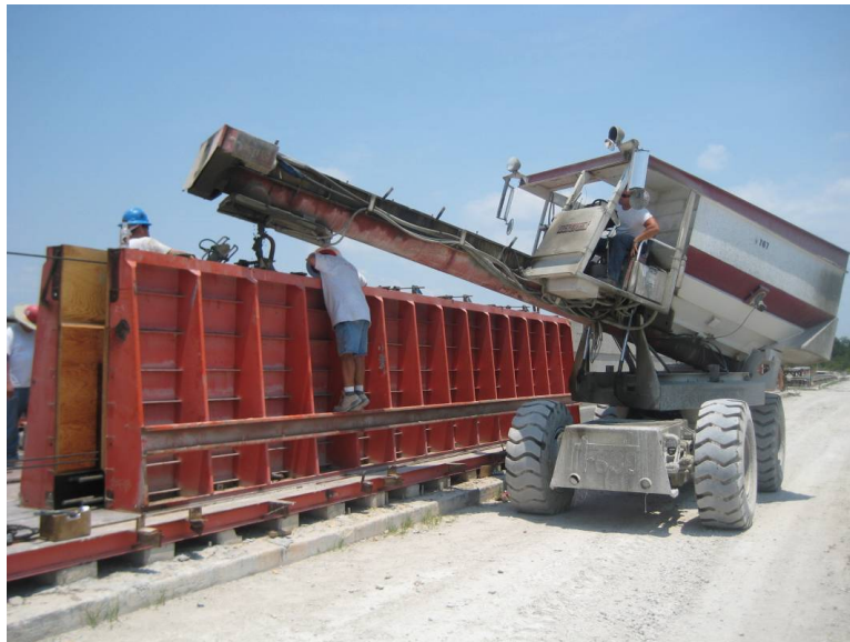
Figure 10.3. Placing concrete in the precast segment formwork
