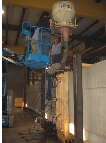
Figure 10.11. Placing concrete into the closure strip formwork
