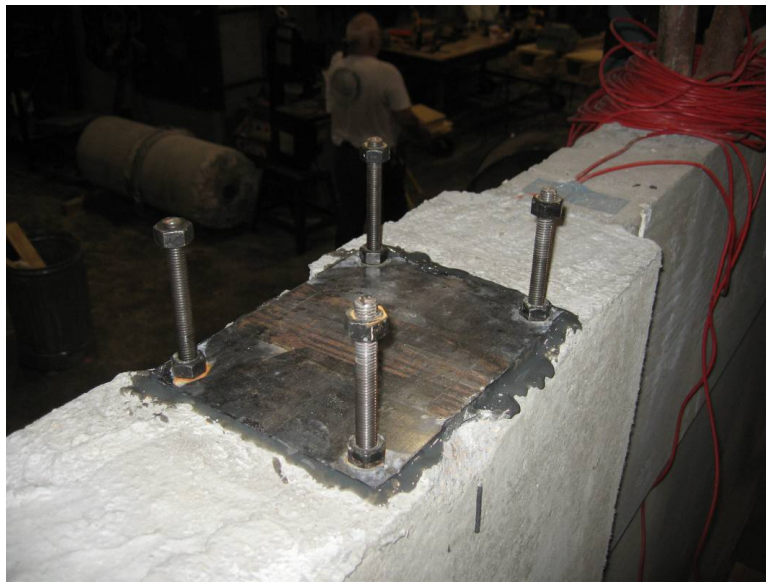
Figure 10.12. Embedded steel plate at top surface of closure strip
