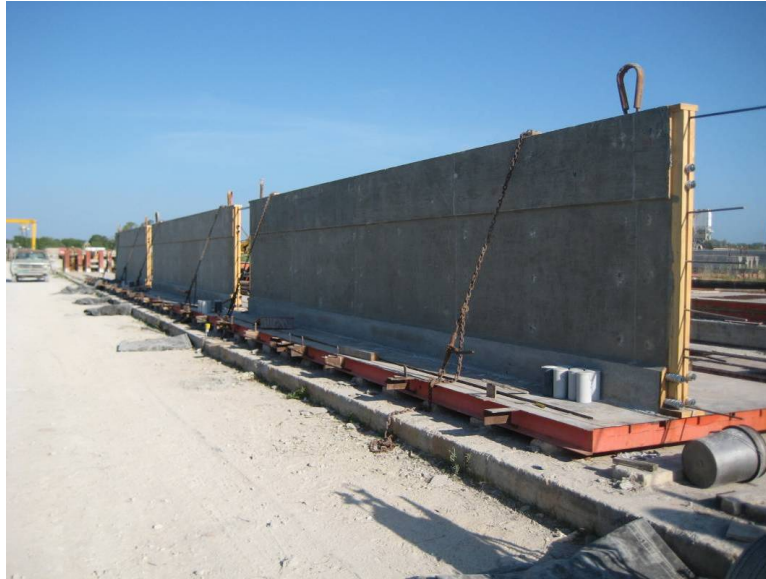
Figure 10.6. Precast segments after formwork removed at Dura-Stress
