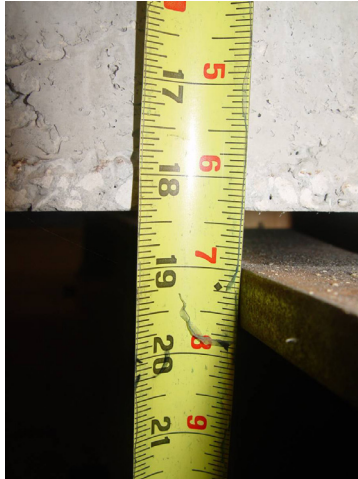
Figure 10.27. Camber measurement at midspan of test girder immediately after completion of post-tensioning
