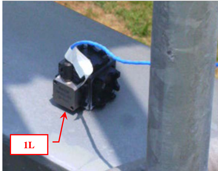
Figure 8-2. Accelerometer 1L measuring the upright in the longitudinal direction normal to traffic
