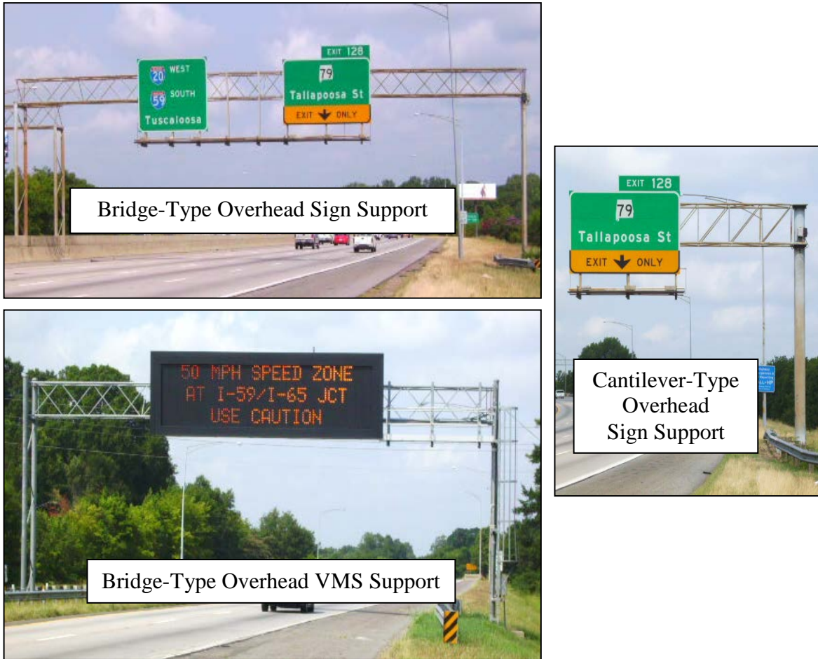
Figure 12-1. Highway overhead support structures with different configurations, sizes and shapes
