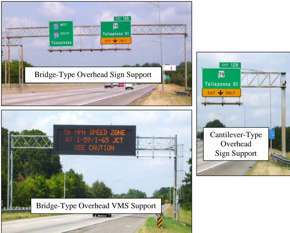
Figure 11-1. Highway overhead support structures with different configurations, sizes and shapes
