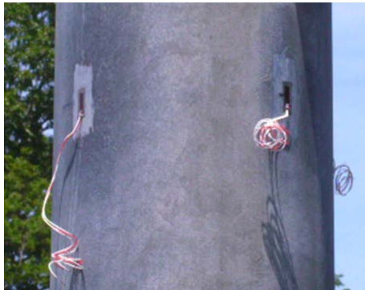
Figure 5-2. Uncovered uni-axial strain gauges attached to the upright post at location 1
