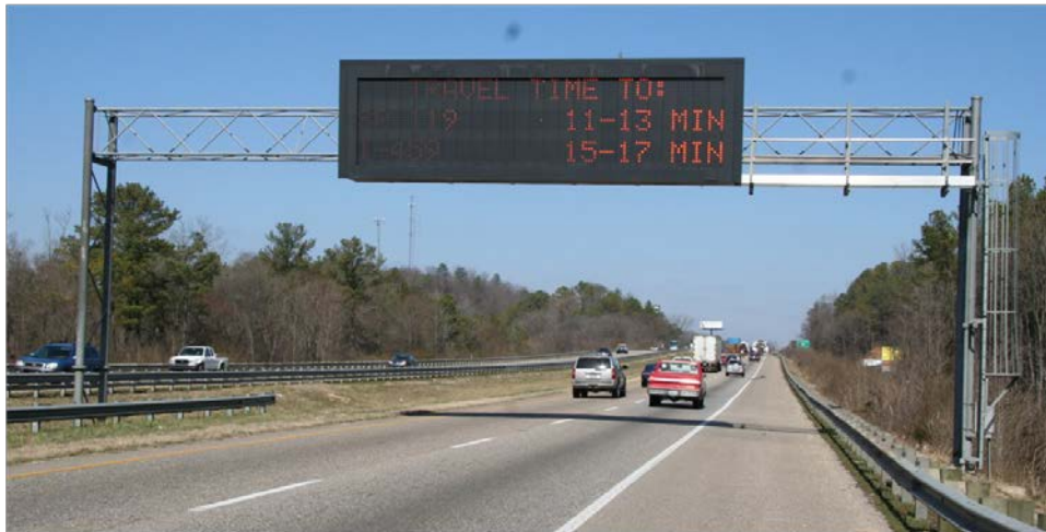
Figure 4-1. Picture of the bridge-type VMS support structure selected for field measurement
