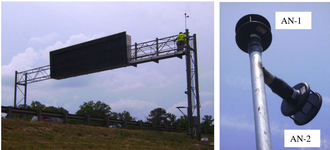
Figure 5-8. Pictures of the anemometers and extension placed 4 ft (1.22 m) above the upright
