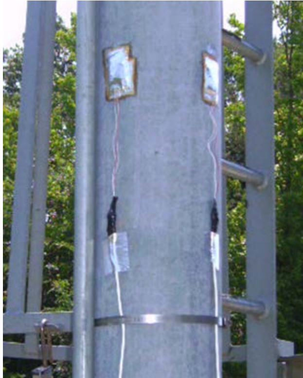
Figure 5-3. Protected uni-axial strain gauges attached to the upright post at location 2
