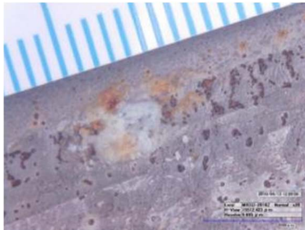
Figure 18 : Pits and corrosion product at ribbed regions of an in-situ SRAP specimen after ~300 days of exposure. 1 mm markers.
