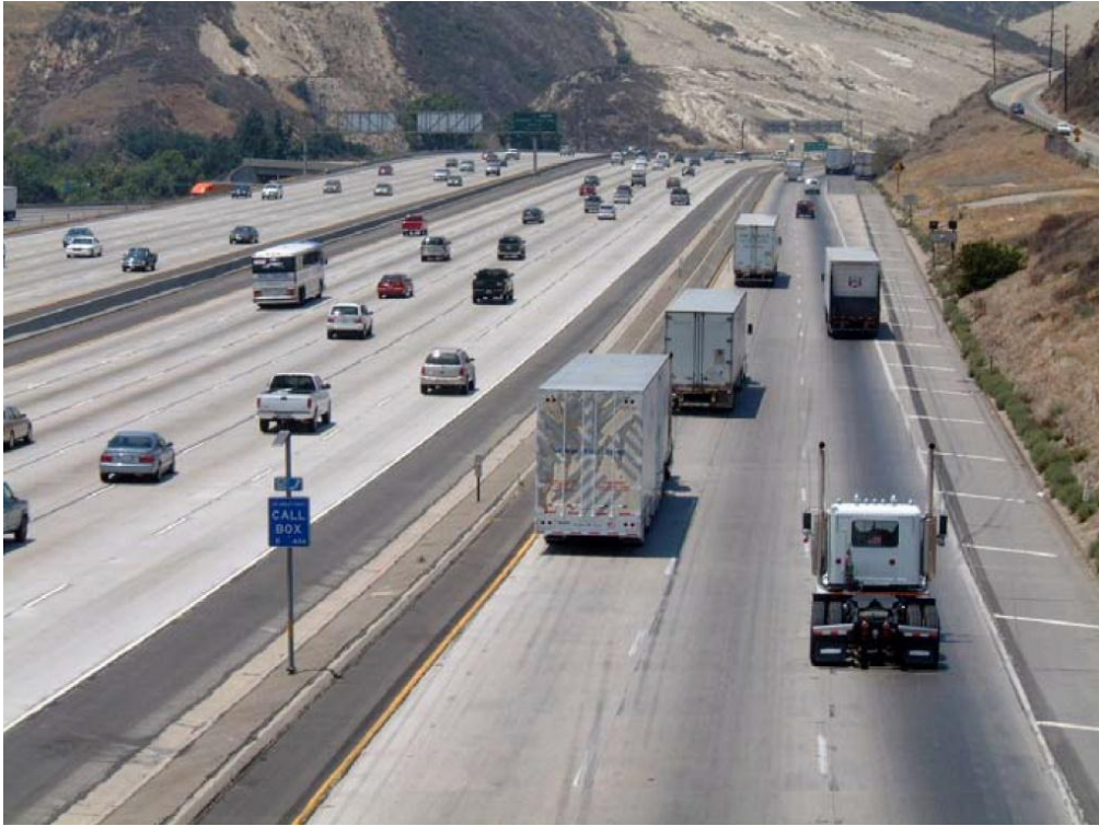
Source: Managed Lanes Handbook (23) Figure 4.1 An Exclusive Truck Roadway, Los Angeles, California
