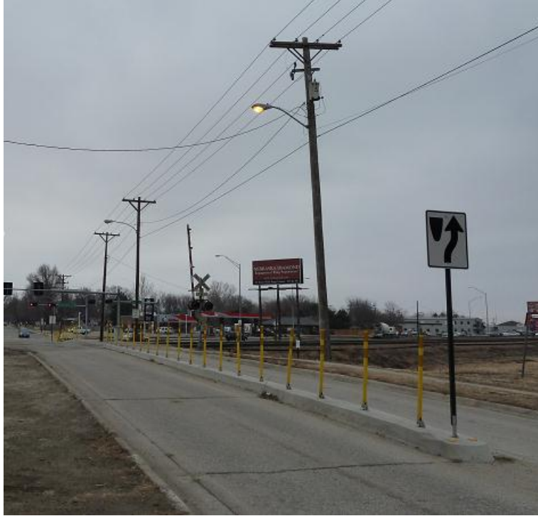
Figure 5.1 Installation of Median Barrier on Raised Concrete Curb at an HRGC
