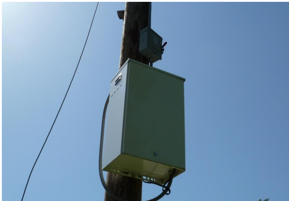
Figure 3.4 Digital Video Recorders (DVR) Housed in Metal Box
