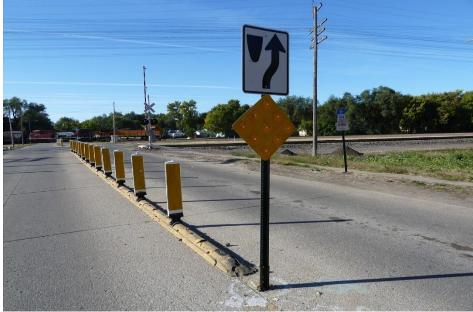
Figure 3.12 Barrier Condition after Maintenance in 2011
