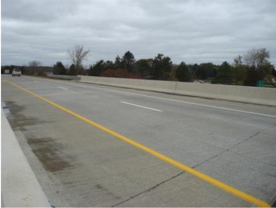
Figure 33. Bridge deck surface
