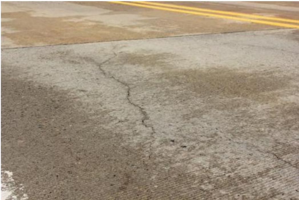
Figure 125. Longitudinal cracking
