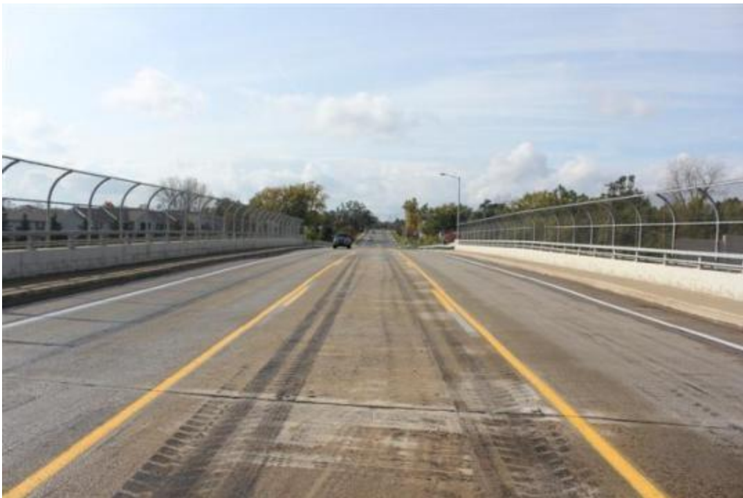
Figure 142. Bridge deck overall view
