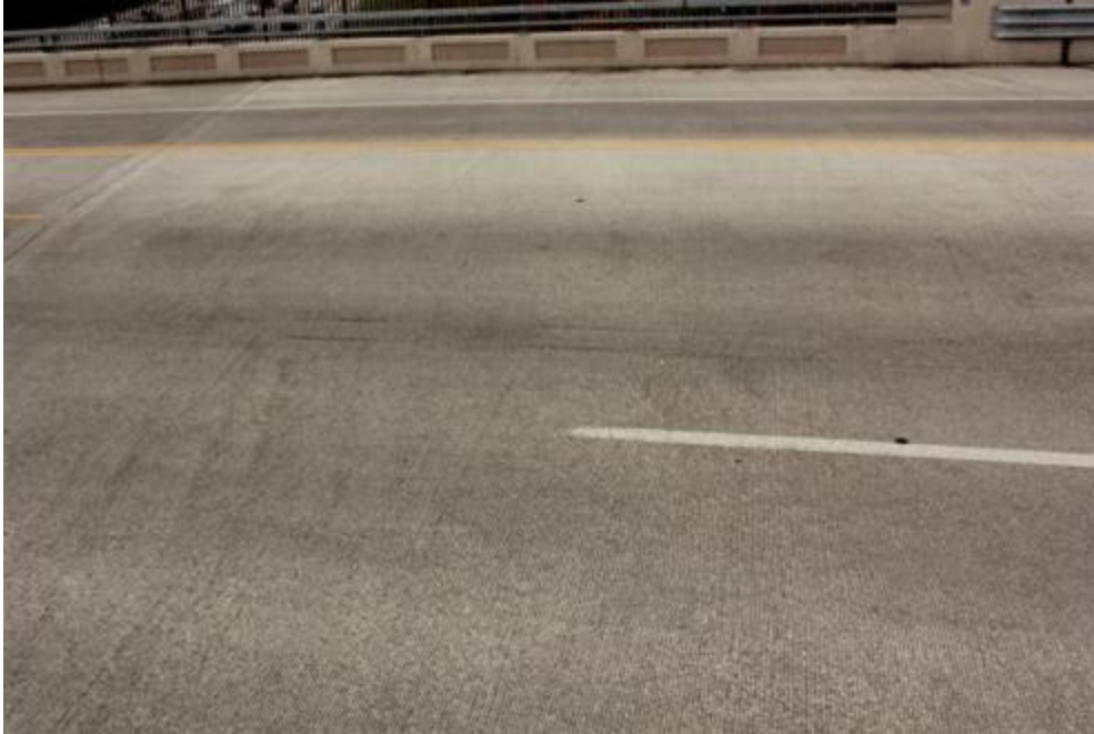
Figure 96. Bridge deck surface
