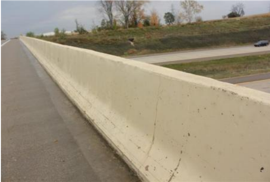
Figure 118. Cracking in barrier wall (typical)
