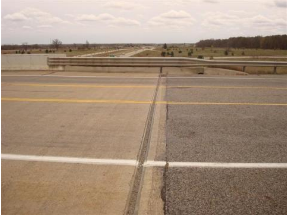
Figure 23. Bridge expansion joint and sleeper slab
