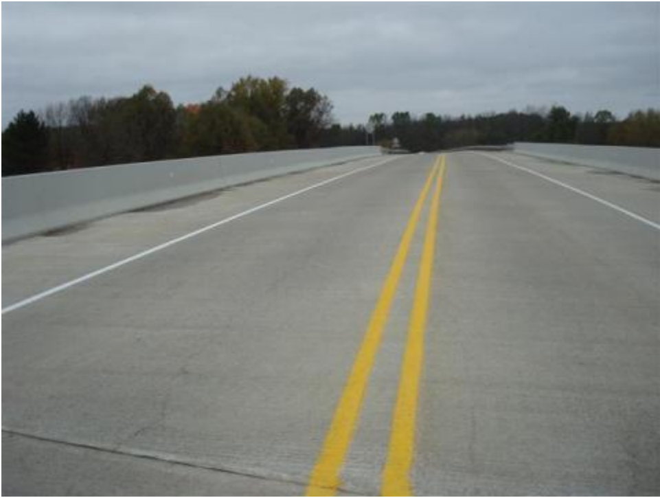
Figure 40. Bridge surface overall view (note longitudinal cracks)
