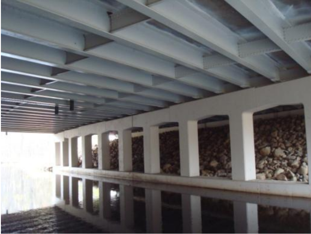
Figure 46. Bridge underside (note no SIP metal forms were used)
