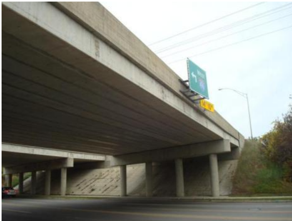
Figure 5. Overall Bridge View
