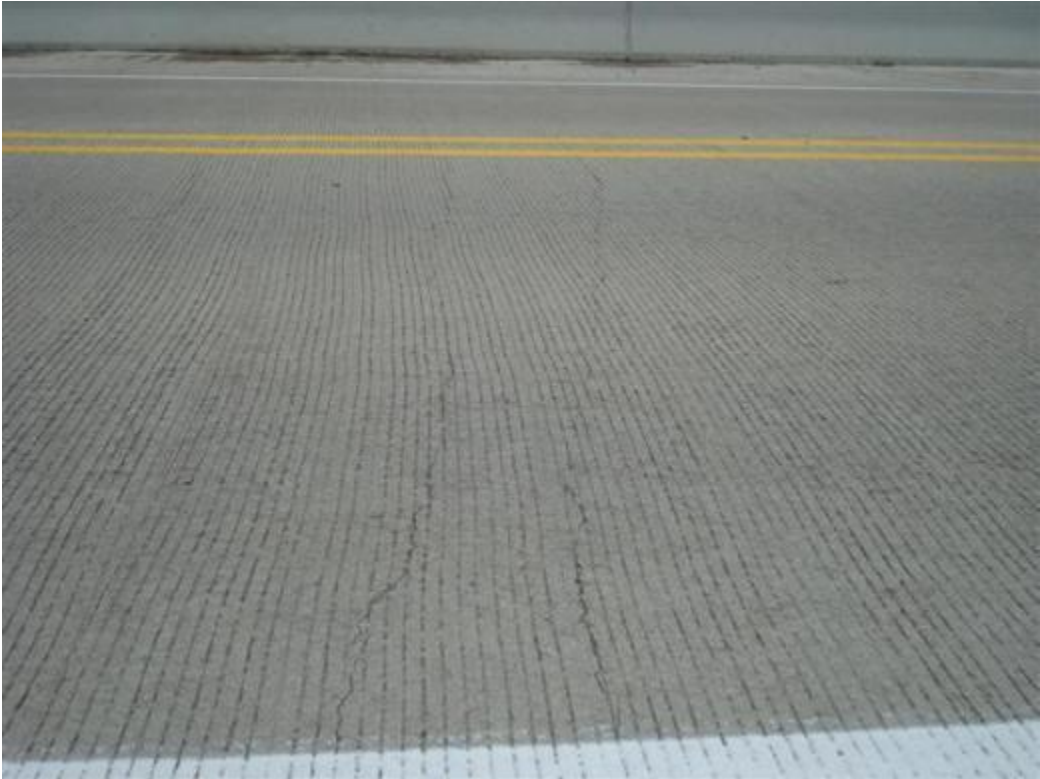
Figure 40. Bridge surface overall view (note longitudinal cracks)
