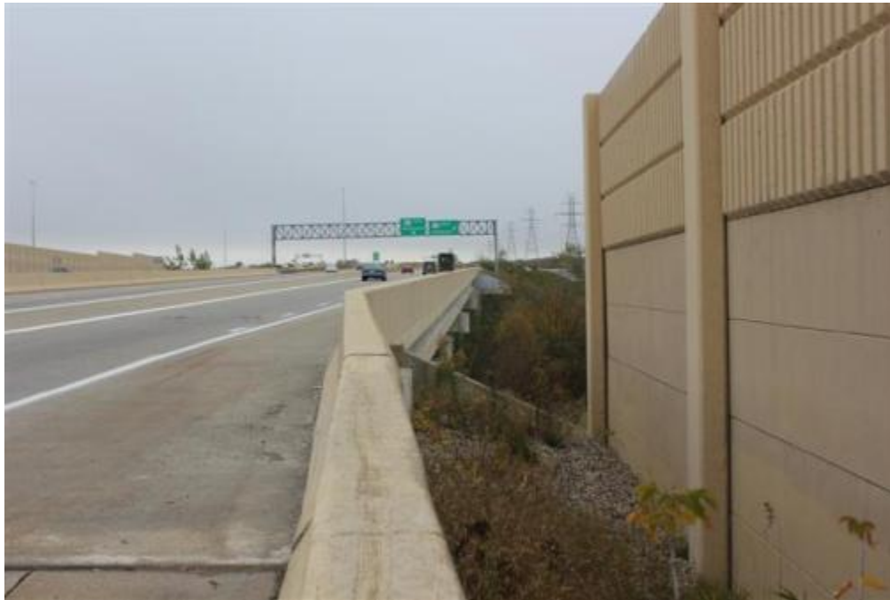
Figure 97. Bridge overall view
