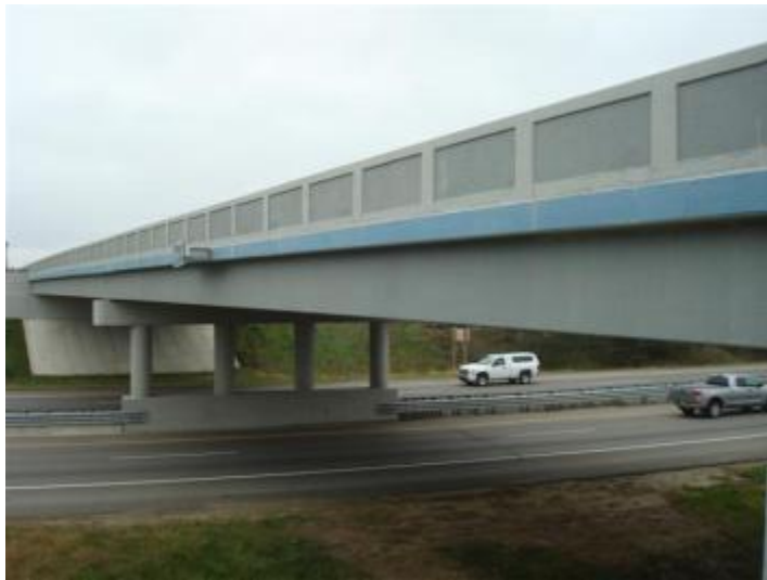
Figure 35. Bridge overall view
