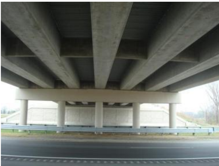
Figure 73. Connection at the abutment (note that beam is not cast into abutment)
