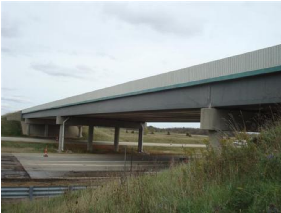
Figure 19. Bridge overall view
