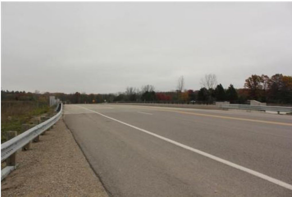
Figure 61. Bridge overall view
