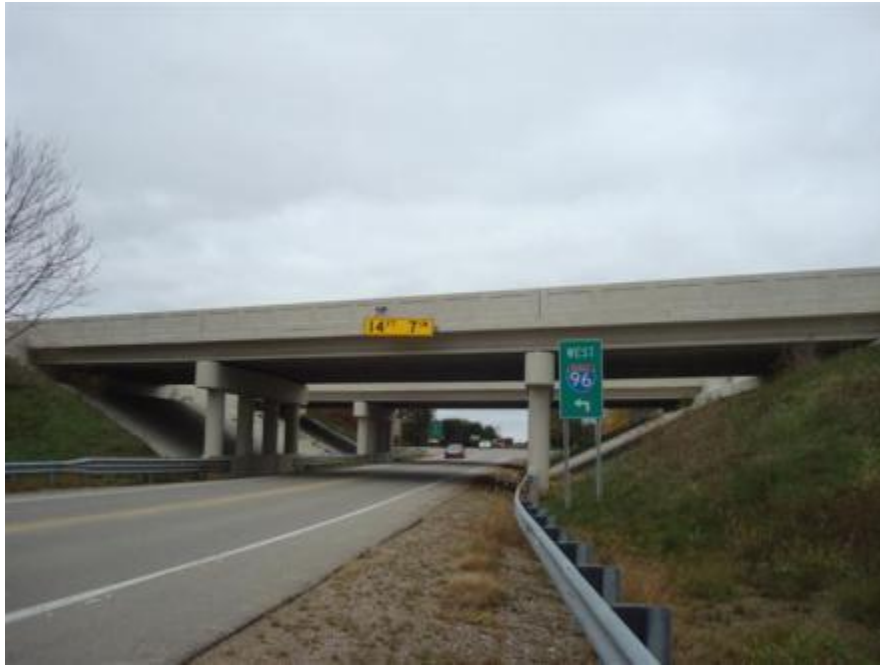
Figure 29. Overall bridge view
