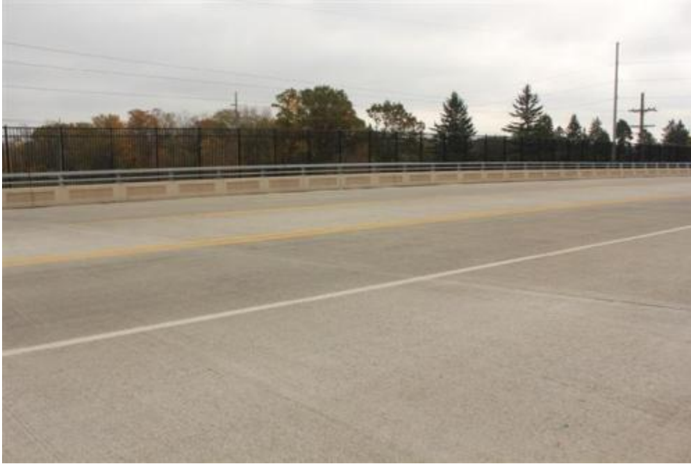
Figure 92. Bridge surface view
