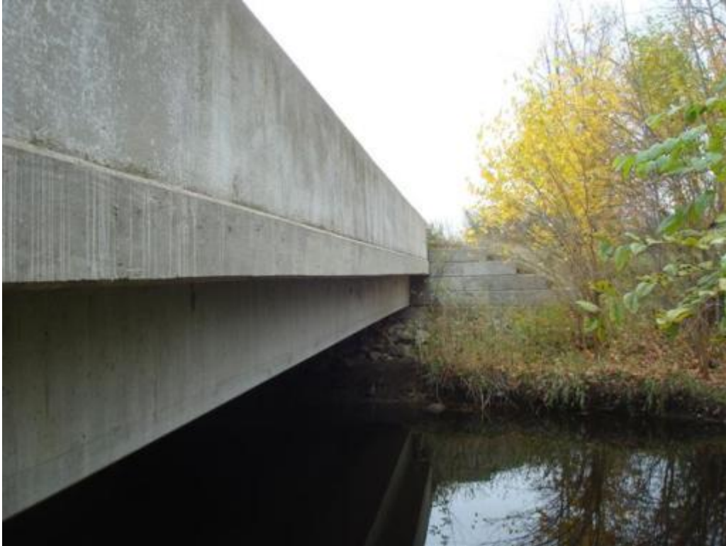
Figure 10. Bridge overall view
