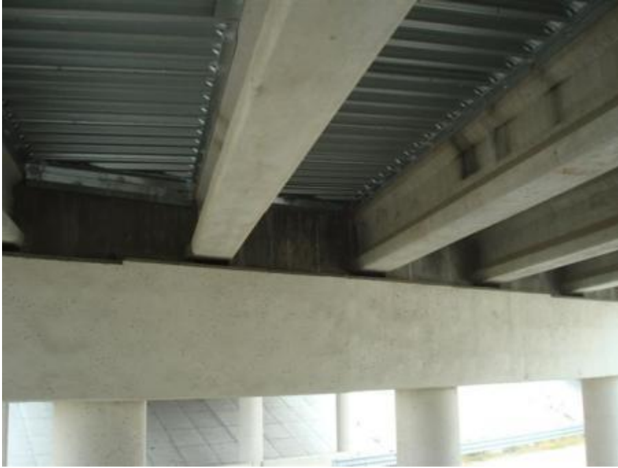
Figure 31. Bridge deck underside
