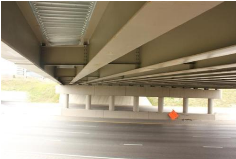
Figure 63. Bridge underside overall view
