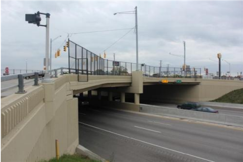
Figure 115. Bridge overall view
