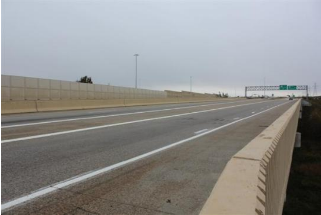
Figure 103. Bridge deck surface overall view
