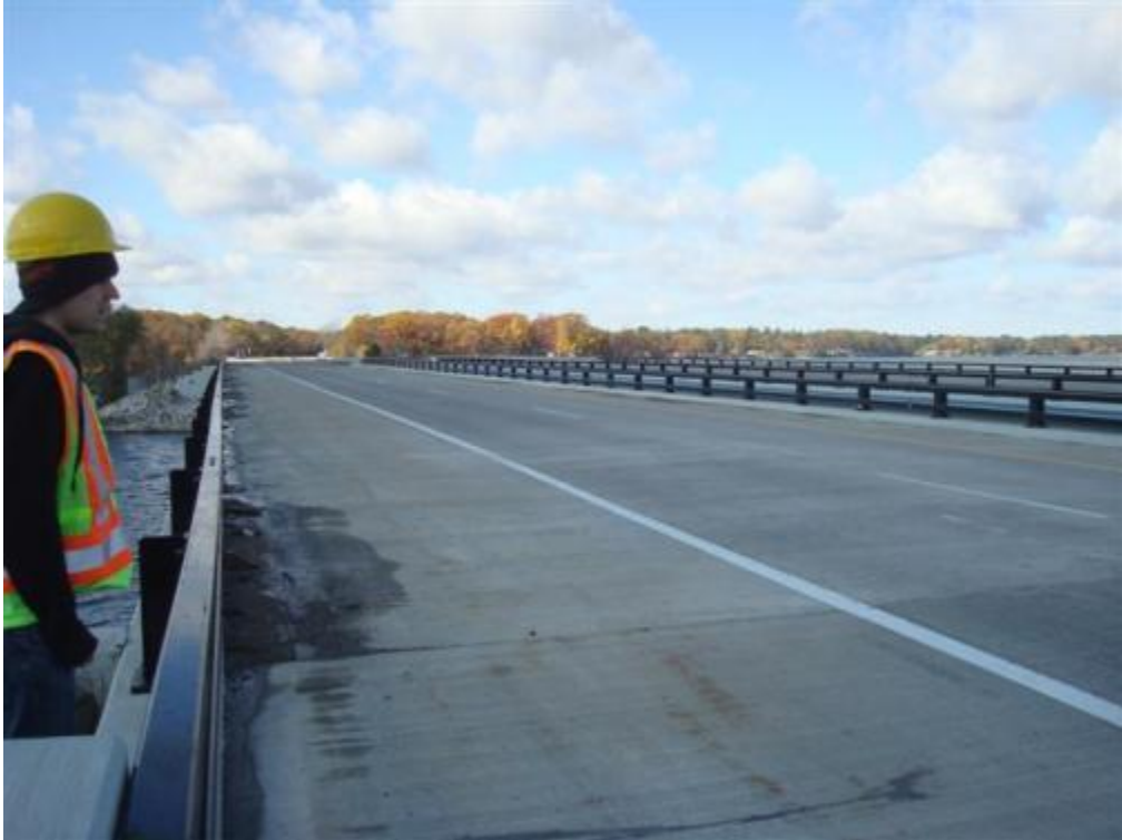
Figure 54. Deck approach slab and expansion joint (some longitudinal cracking)
