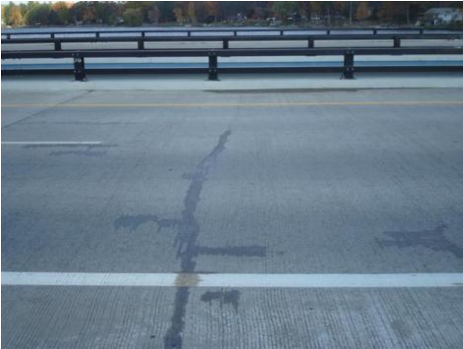
Figure 59. Additional transverse cracking at pier 2, as well as some longitudinal cracking
