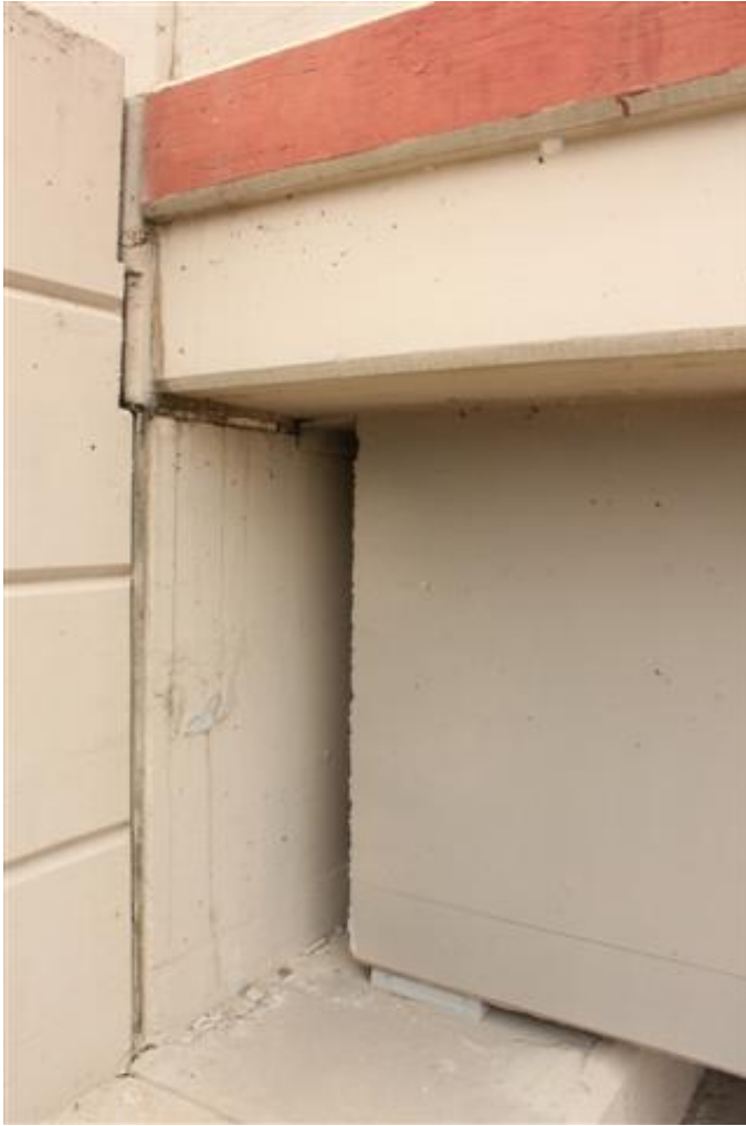
Figure 73. Connection at the abutment (note that beam is not cast into abutment)
