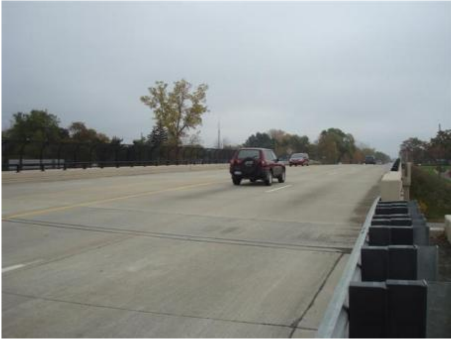
Figure 85. Bridge surface overall view
