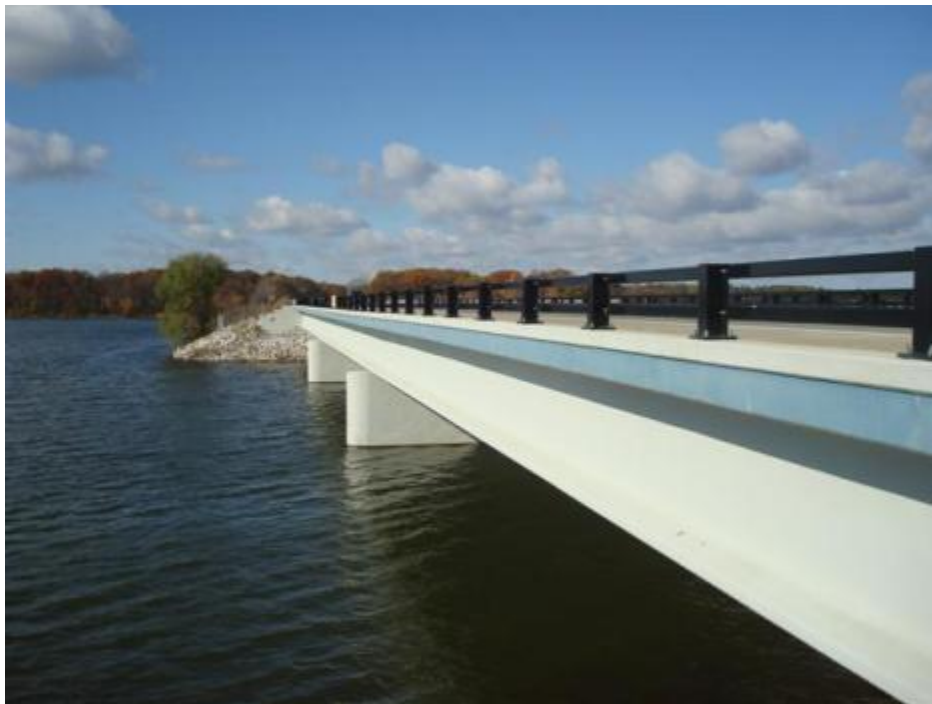
Figure 51. Overall Bridge View (Eastbound side)
