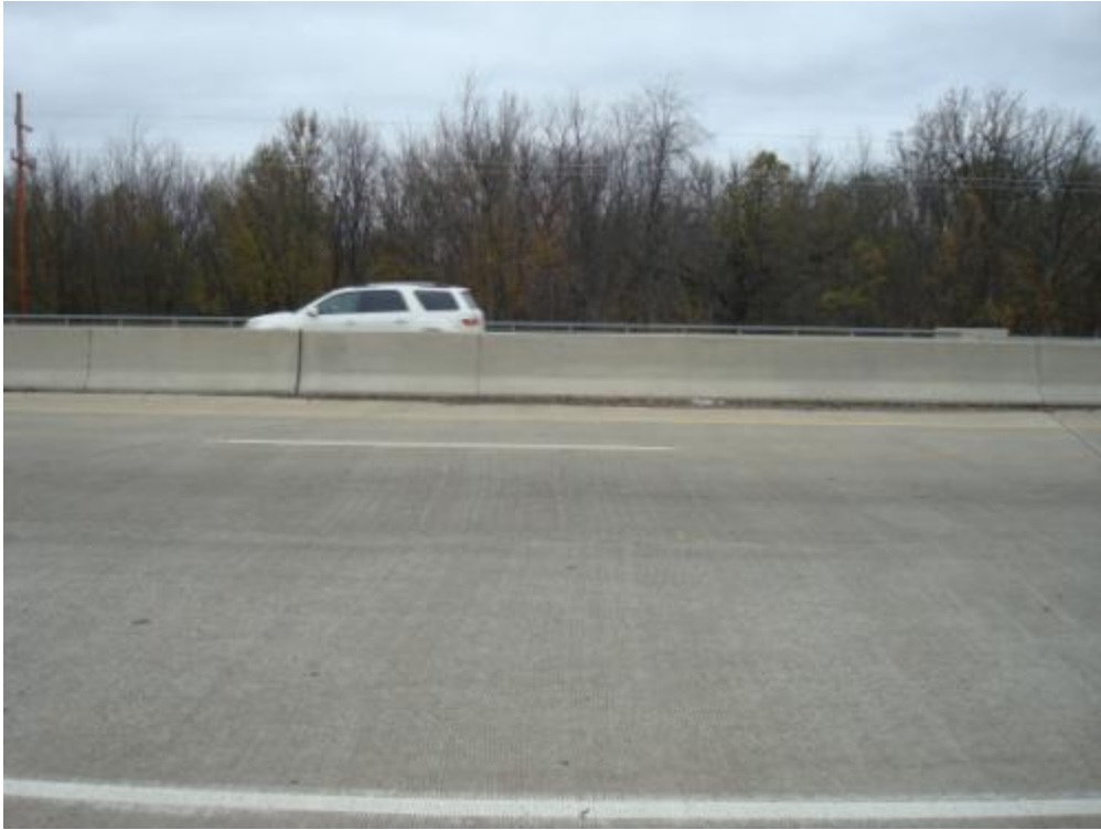
Figure 49. Bridge deck surface (no notable cracks)
