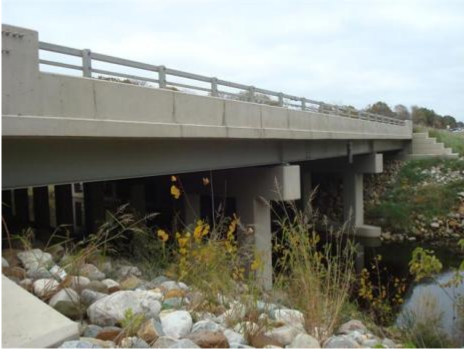
Figure 44. Bridge overall view
