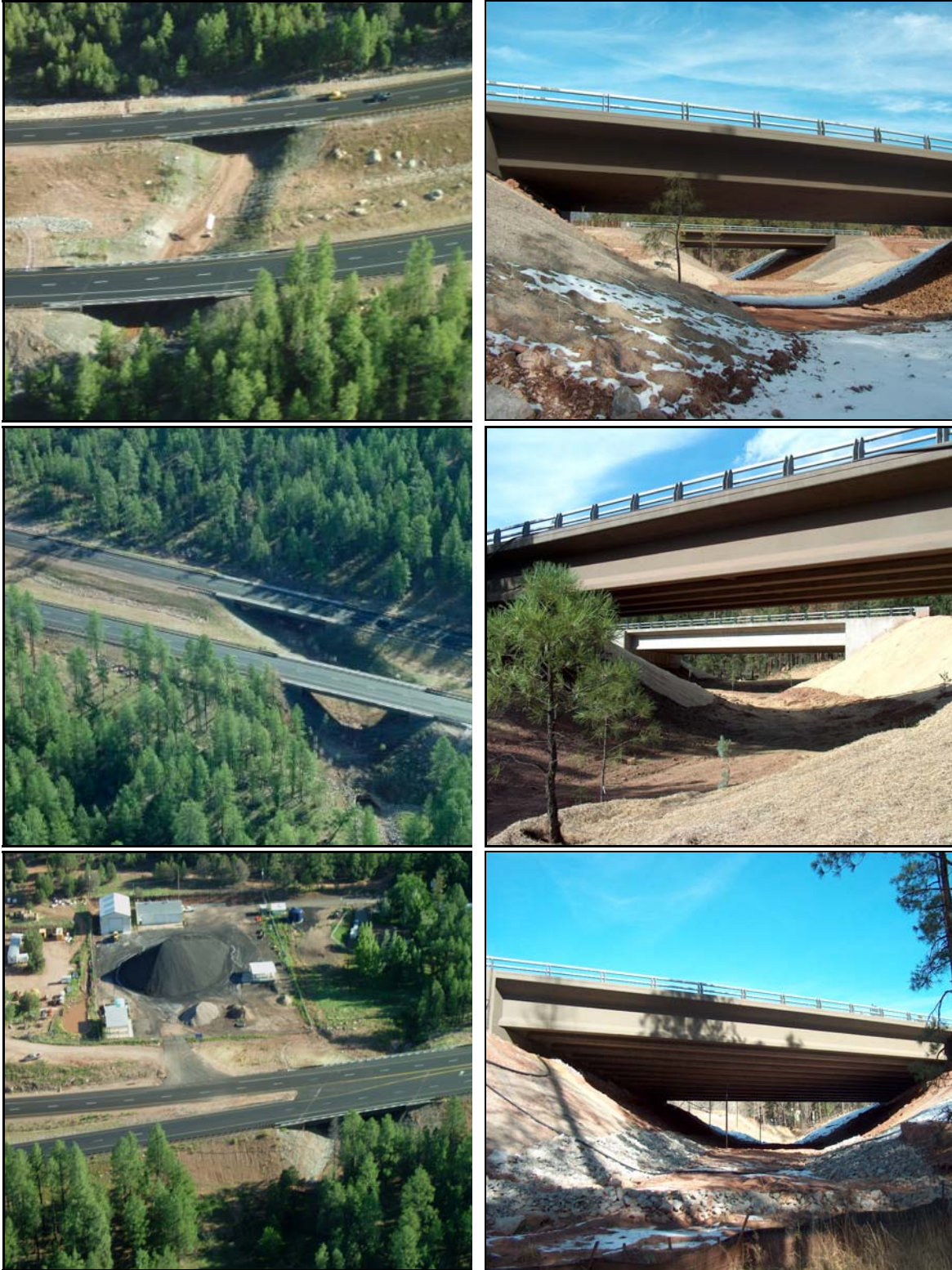
Figure 8. Aerial and Ground Photographs of SR 260 Underpasses, Including Pedestrian-Wildlife Underpass (Top), Wildlife 2 Underpass (Middle), and Wildlife 3 Underpass (Bottom).
