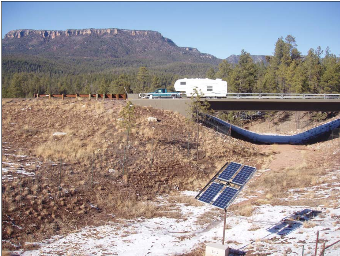
Figure 3. SR 260 Study Area at the Pedestrian-Wildlife Underpass on the Christopher Creek Section, with Mogollon Rim Escarpment (Background) and Solar Panels for Powering Video Camera Surveillance System (Foreground).
