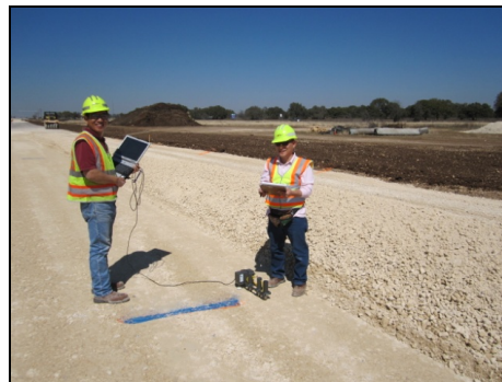
Figure 2.4. PSPA Testing on US 183 Flex Base.
