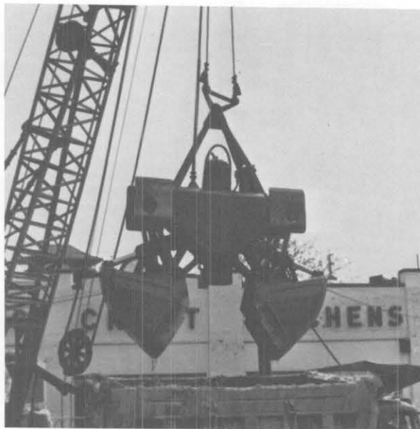
2'6" x 14'0" Hydraulic Clam Shell
