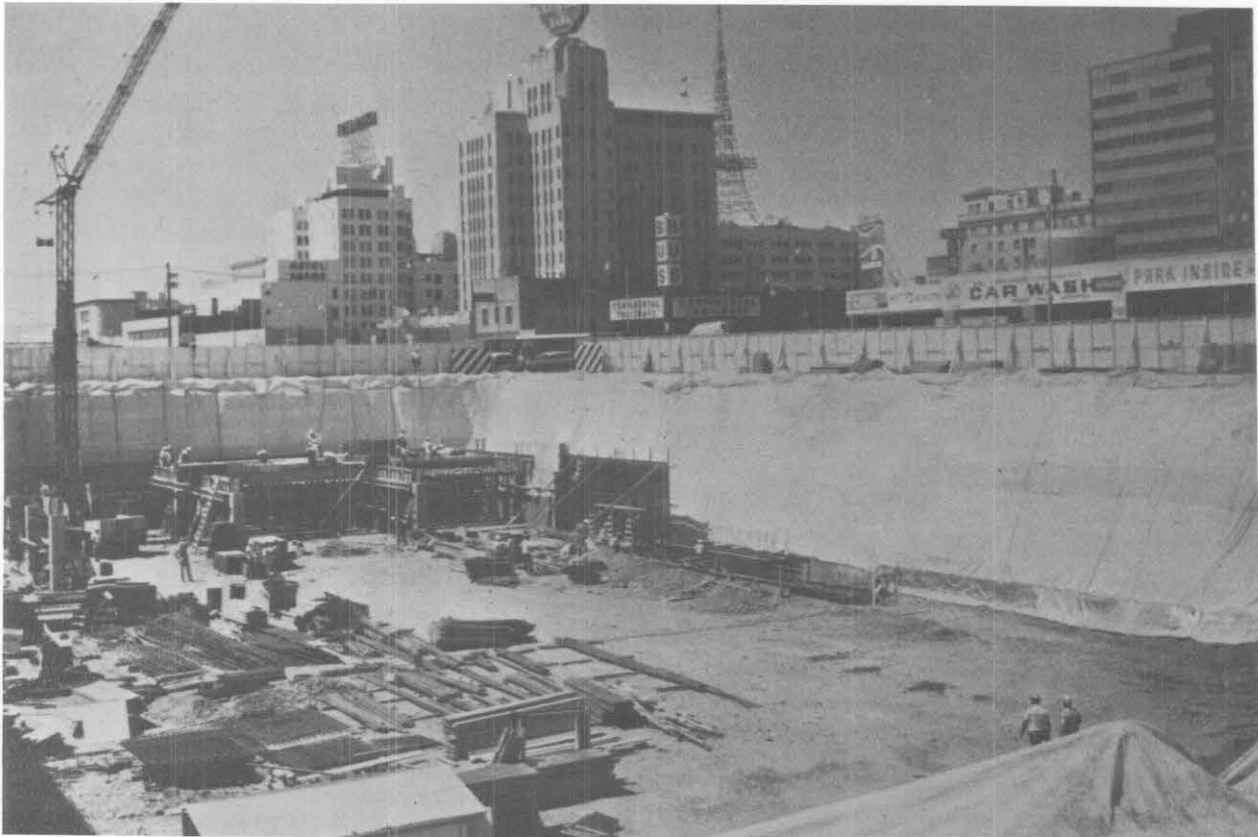
Figure 140. Freeze wall surrounding open excavation. (Courtesy of Terrafreeze Corporation).
