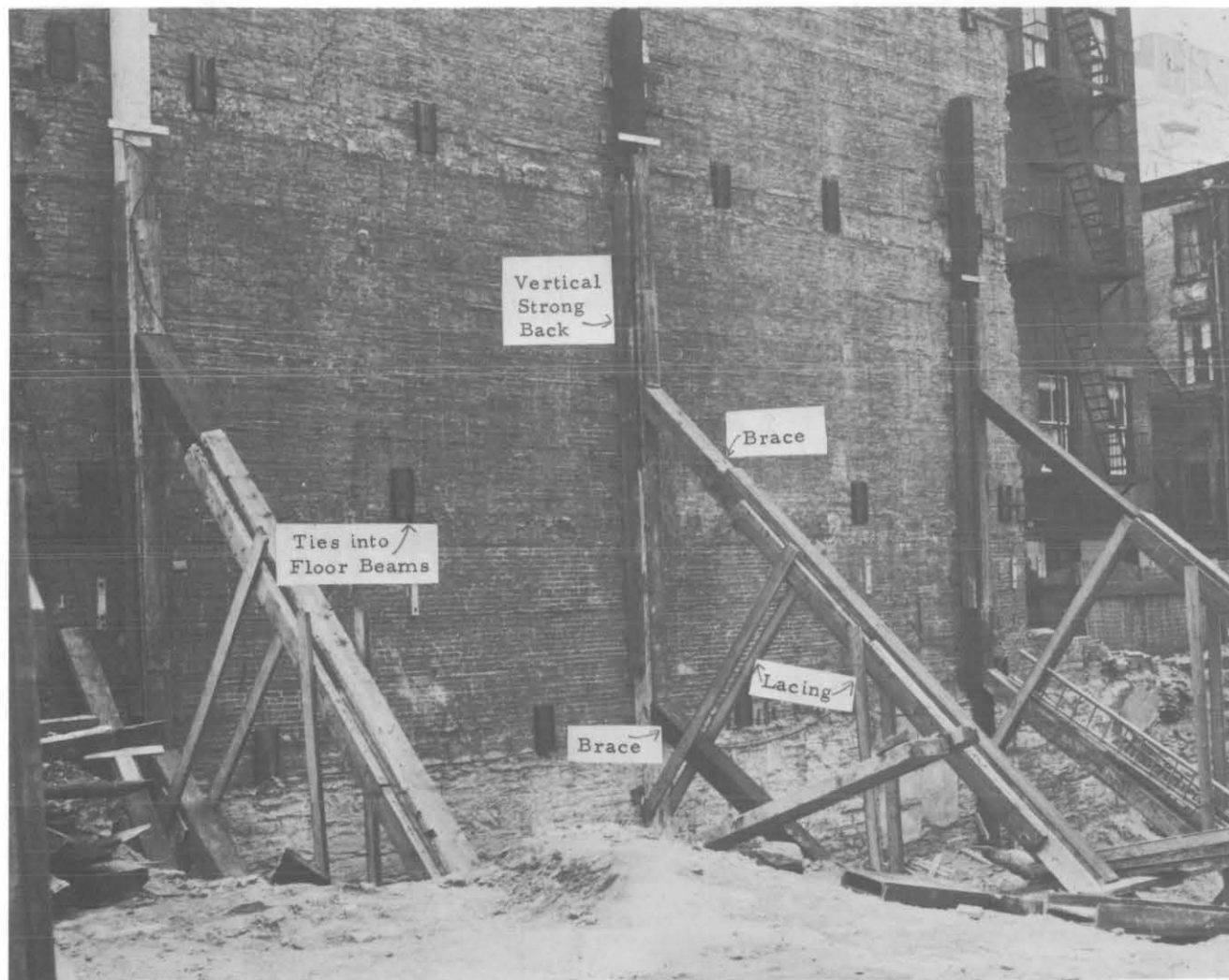
Figure 124. Lateral bracing of wall prior to underpinning. (Courtesy of Spencer, White, and Prentis).
