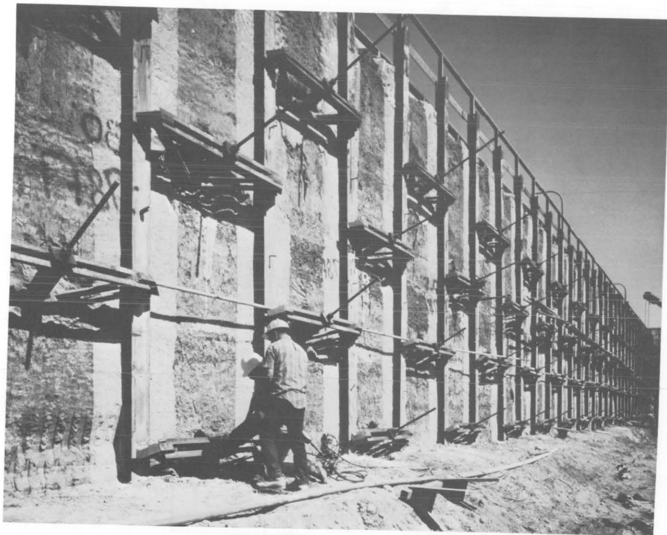
Figure 77. Example of tied-back wall using channel sections as wales. (Courtesy of Hughes Tool Company).
