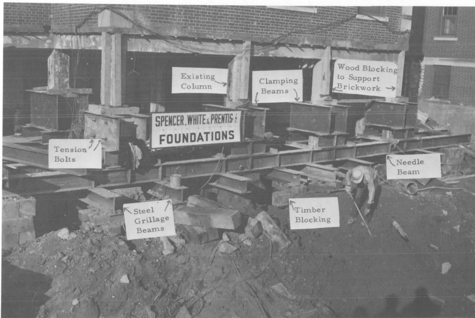
Figure 129. Shoring of concrete columns. (Courtesy of Spencer, White, and Prentis).
