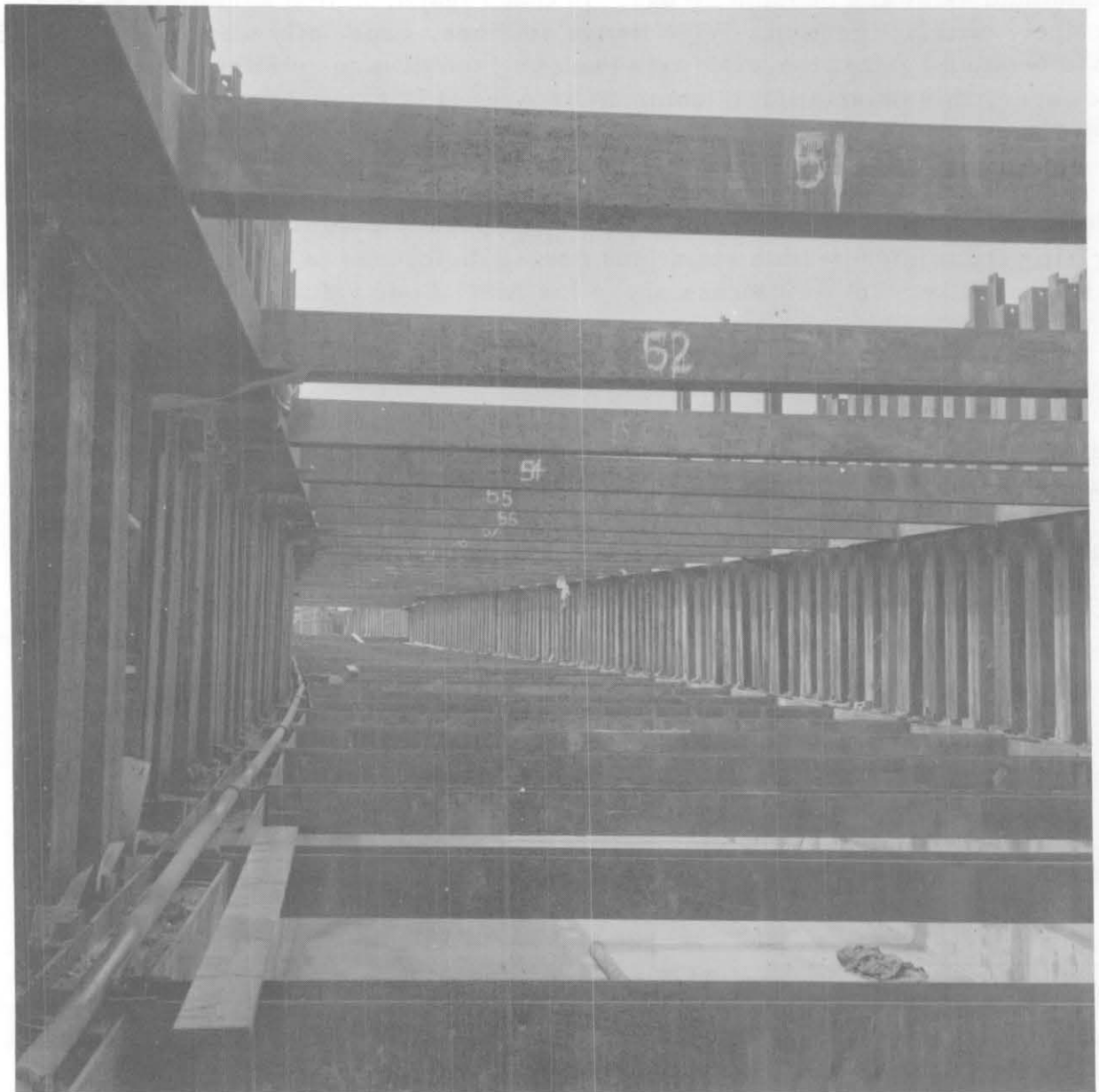
Figure 42. Internal bracing. (Courtesy of Perini Corporation).
