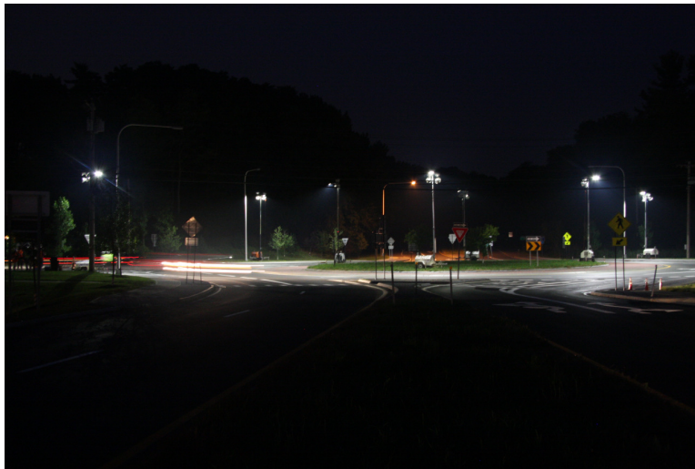
Figure 20. White light streetlight demonstration. Photo taken from Rt. 85 entrance to roundabout.
