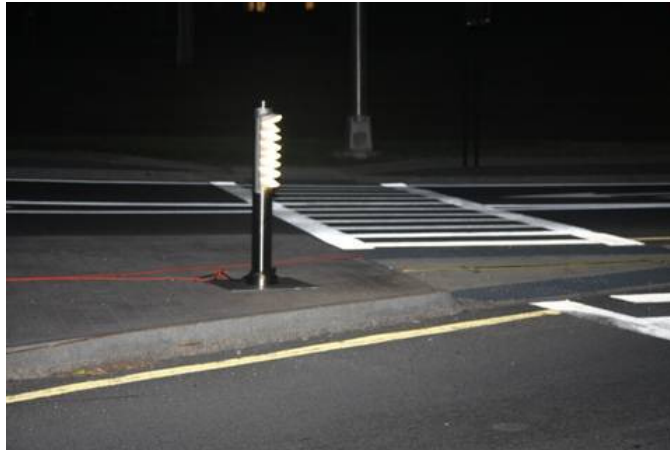
Figure 31. Pedestrian bollard luminaire with louvers.
