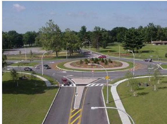
Figure 1. Photograph of a roundabout in New York State, showing the use of pole-mounted lighting (from NYSDOT website).
