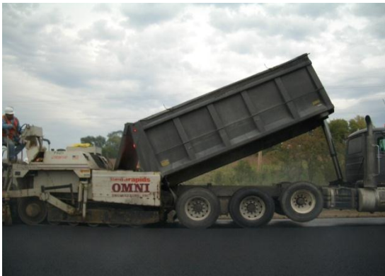
Figure 4.6 Direct Dump between Truck and Paver
