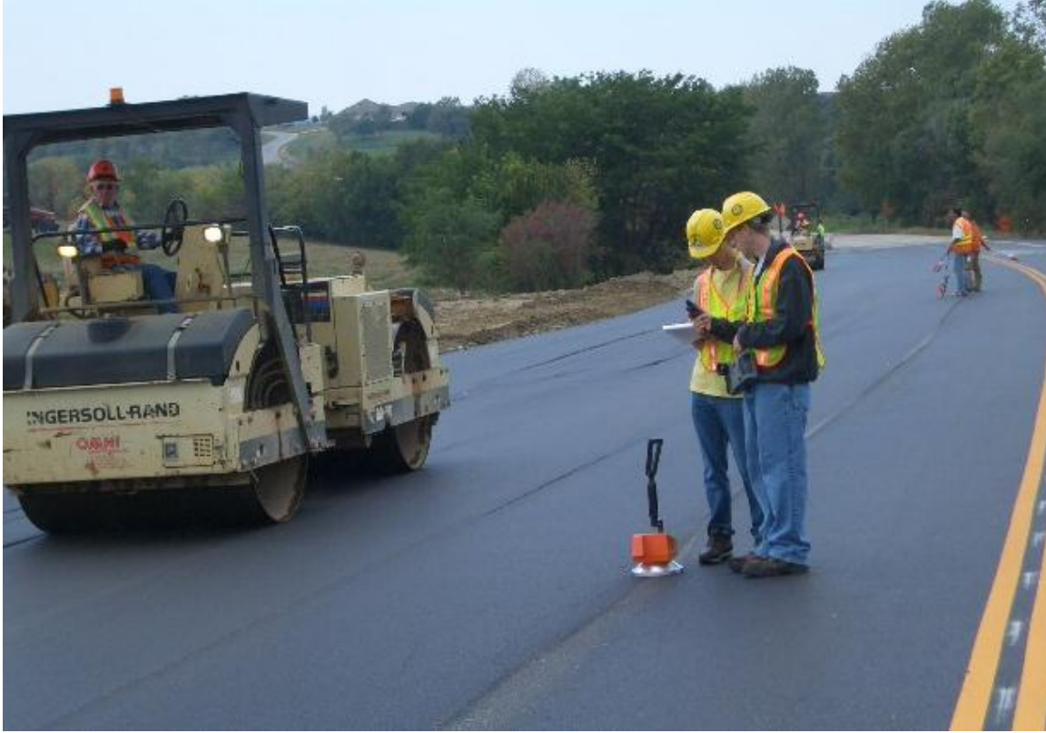
Figure 3.3 Taking PQI Density Readings Onsite
