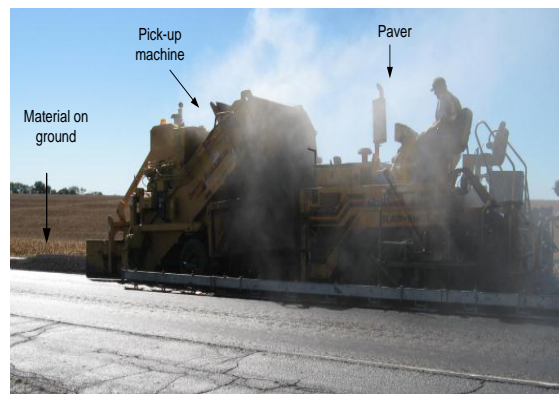
Figure 4.7 Pick-up Machine with Paver
