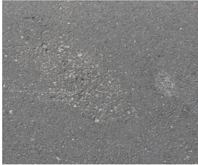
Figure 5.4 Observed Material Segregation
