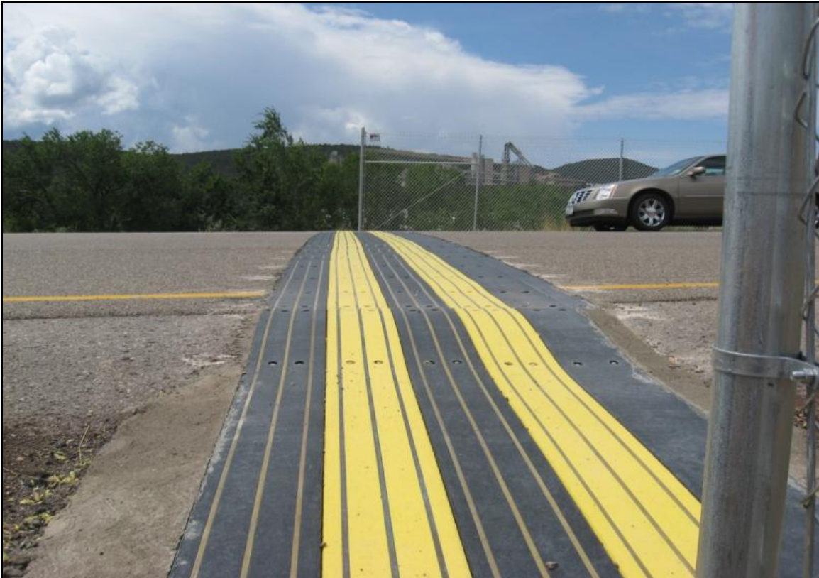
Figure 28. An Electrified Barrier Installed in the Pavement to Prevent Wildlife from Breaching the Fenced Corridor at the Fencing Terminus. This Mat was Installed on I-40 Off-Ramps in New Mexico.
