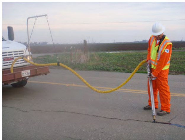
Figure 37. Manual Sealing Hose and Support Boom
