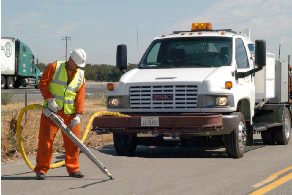
Figure 11. Sealzall In-Lane Sealing
