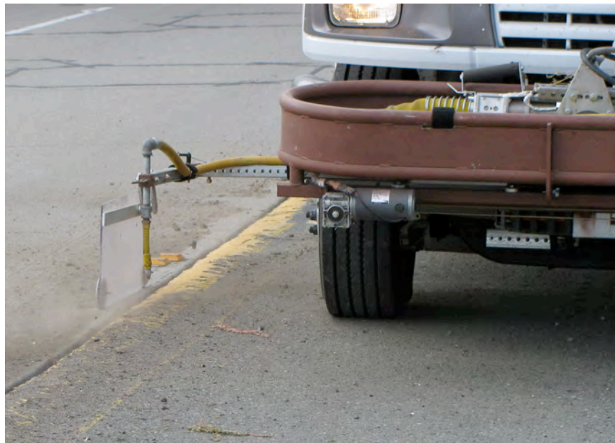
Figure 8. Longitudinal Crack Cleaning
