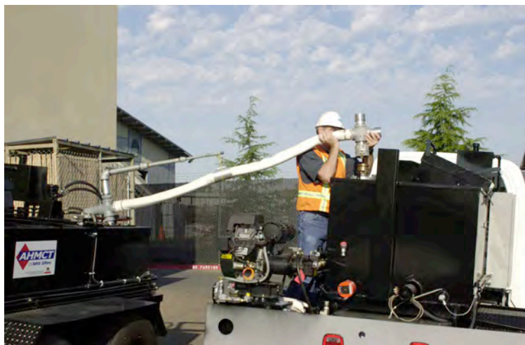
Figure 3. TTLS Sealant Transfer
