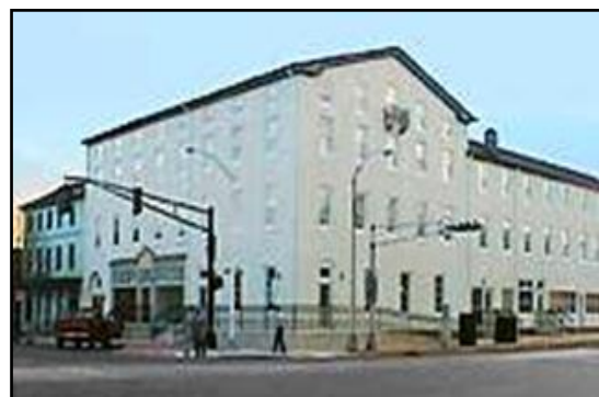
Figure 12. The Metropolitan Inn. Source: DVRPC
