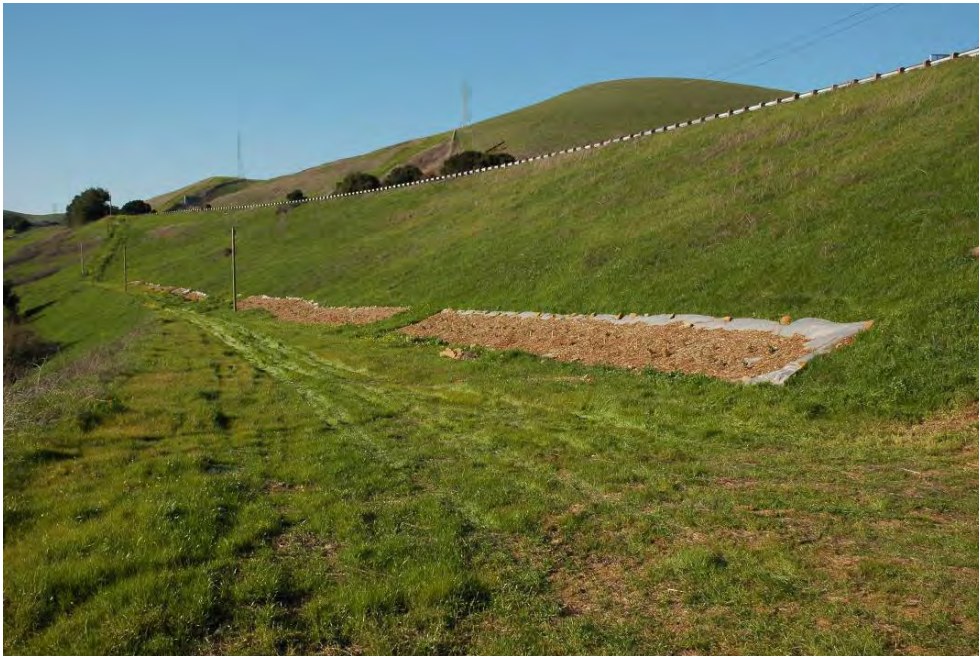
Figure 1. Demonstration plots at CC SR 4 after construction in February 2006.
