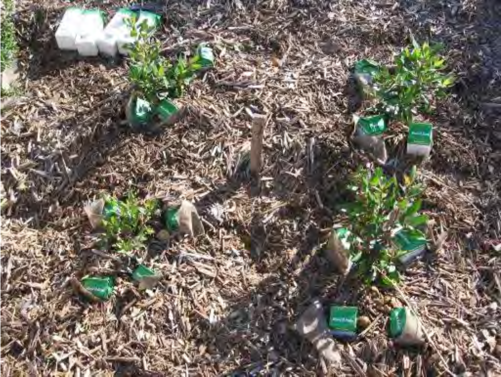
Figure 2. Water retaining gel installation at Contra Costa SR 4
