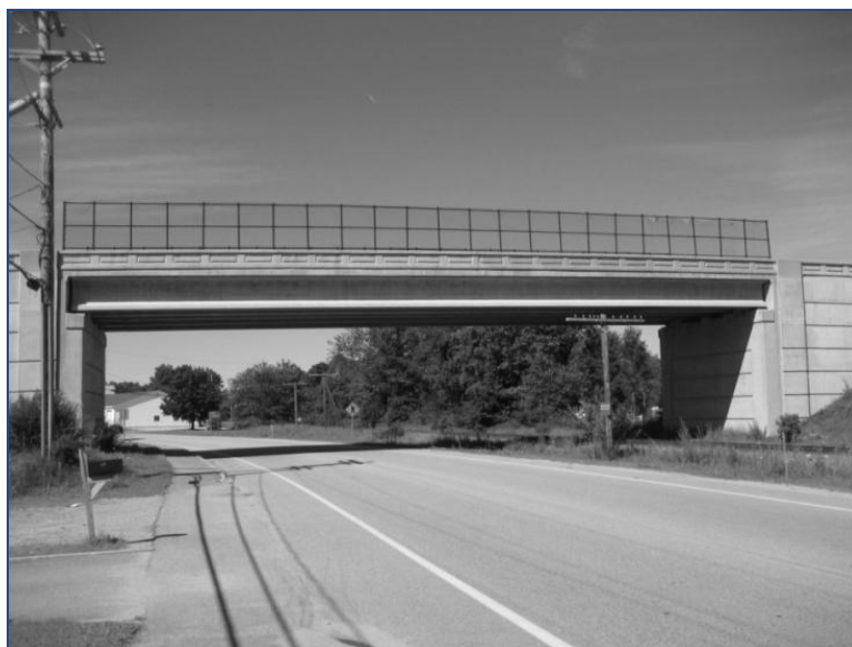
Figure 4: New Rollins Road Bridge, opened in 2000
