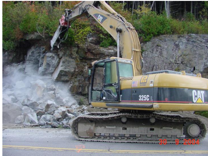
Figure 14 - Track mounted excavator on pavement
