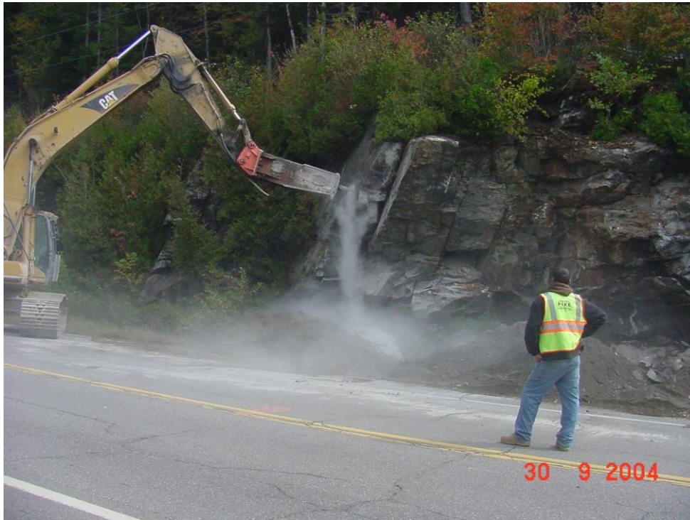
Figure 7 - Hoe-ram breaking up rock
