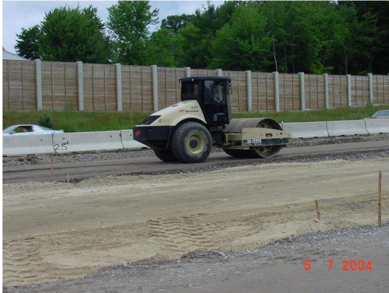
Figure 4 - Vibratory roller compacting base course material
