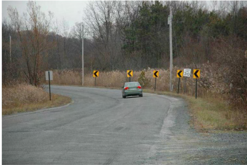
Figure 2-5. Test curve equipped with the modified chevron treatment.
