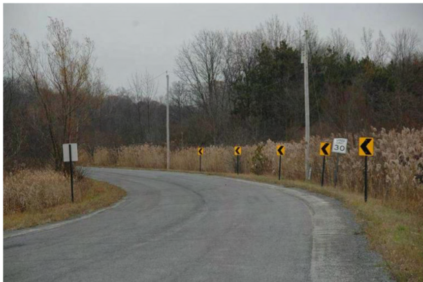
Figure 2-4. Test curve equipped with the conventional chevron treatment.
