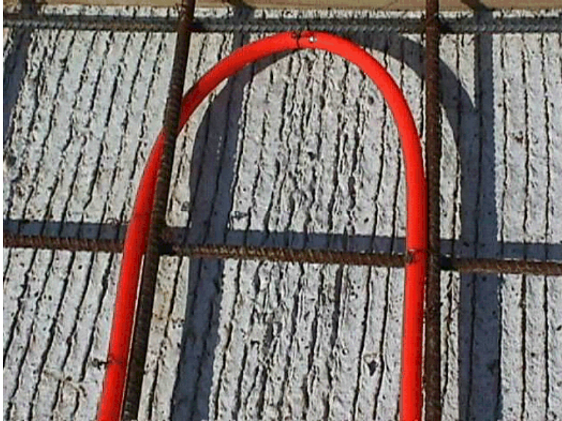
Figure 13-5. Pipe for Heating Bridge Deck.
