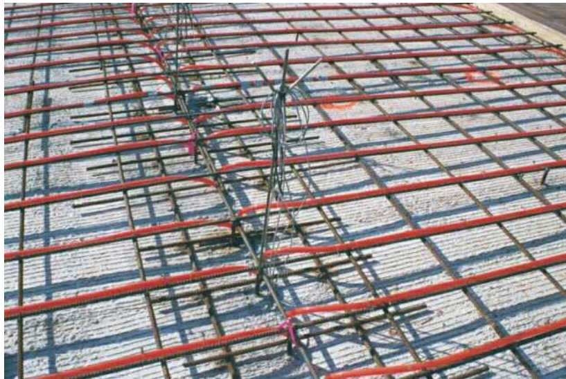
Figure 13-6. Bridge Deck Showing Instrument Wire on Trees.
