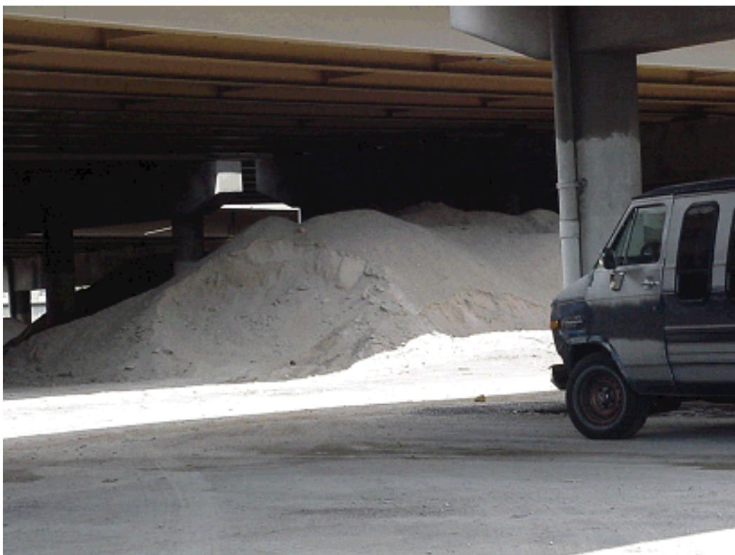
Figure 9-11. Salt Storage under a Bridge Next to Bridge Columns.
