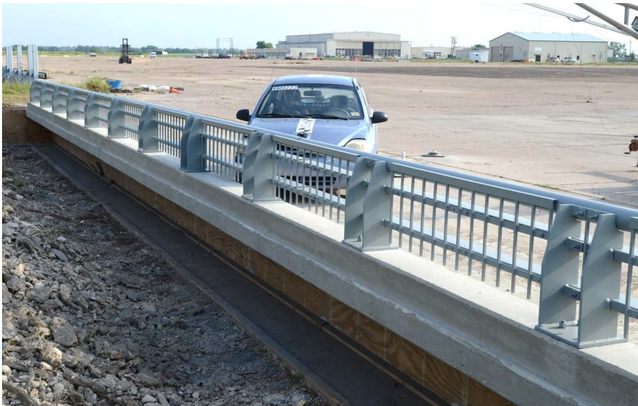
Figure 5.1. Vehicle/Installation Geometrics for Test No. 490022-2.
