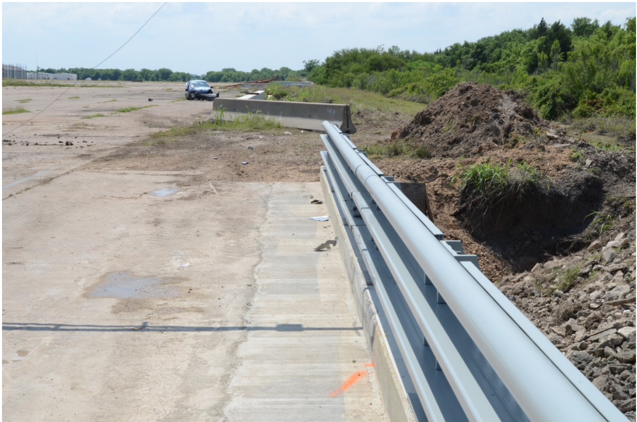
Figure 5.3. Vehicle/Installation after Impact for Test No. 490022-2.
