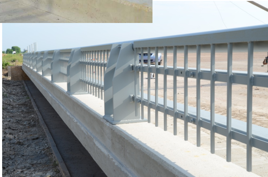
Figure 2.3. TxDOT Picket Rail before Testing.
