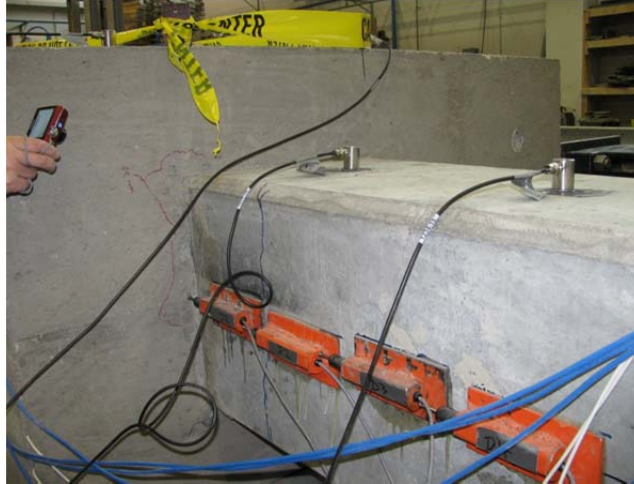
Figure 7.7 Joint Region following Test Completion - Specimen EB-18-1
