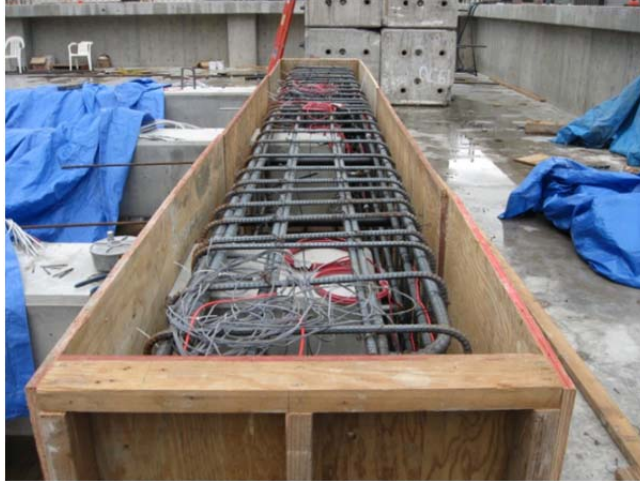
Figure 8.15 Bent Cap Prior to Casting - Three Pile Specimen
