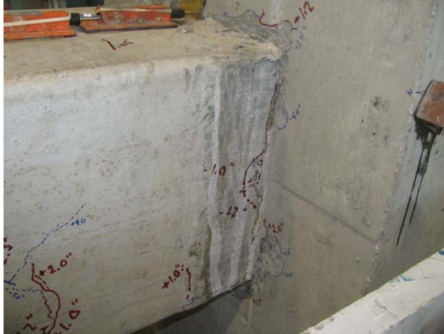
Figure 6.37 Joint Region Following Test Completion - Specimen IB-22-1
