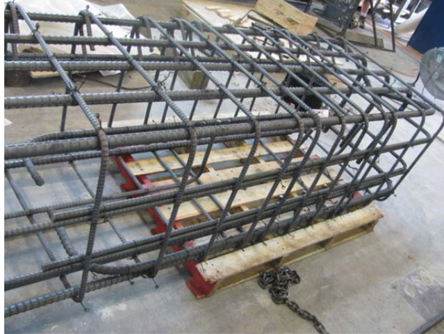
Figure 8.10 Reinforcement Cage, Cantilevered End
