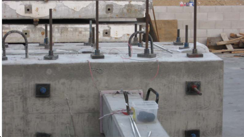
Figure 8.22 Footing Connections - Three Pile Specimen
