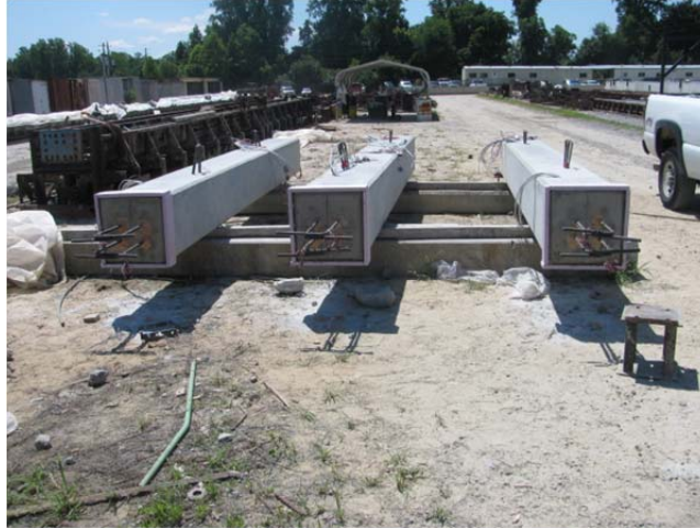
Figure 8.4 Pile Hinge Construction - Three Pile Specimen
