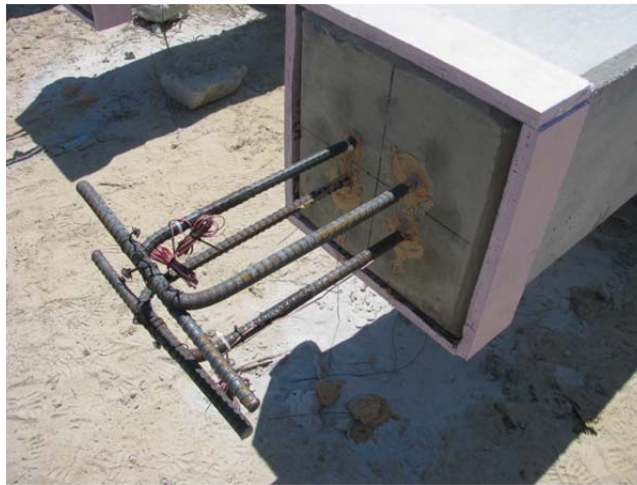
Figure 8.5 Pile Hinge Construction - Three Pile Specimen
