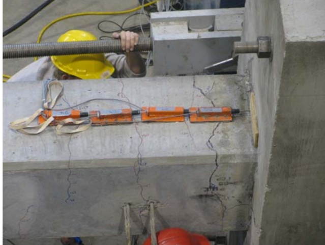
Figure 6.25 Observed Pile Damage - Specimen IB-26-1
