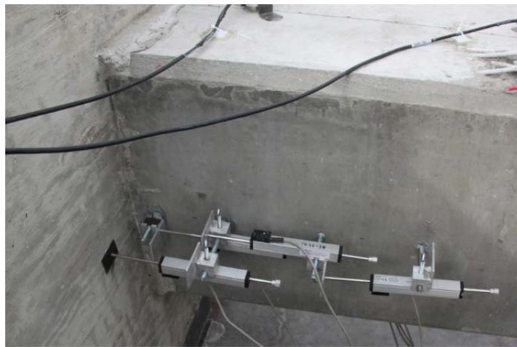
Figure 8.31 Novatecknic Gages - Three Pile Specimen
