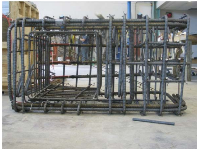
Figure 3.7 Reinforcement Cage - Specimen EB-26-1
