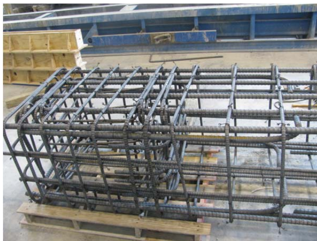
Figure 8.12 Reinforcement Cage, Heavily Reinforced End
