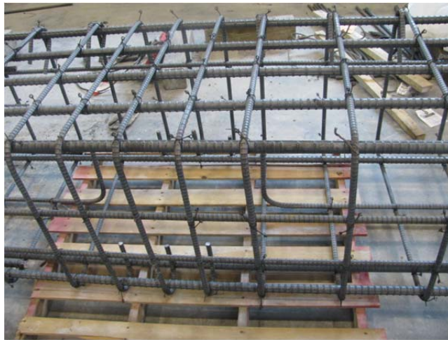
Figure 8.11 Reinforcement Cage, Interior Portion
