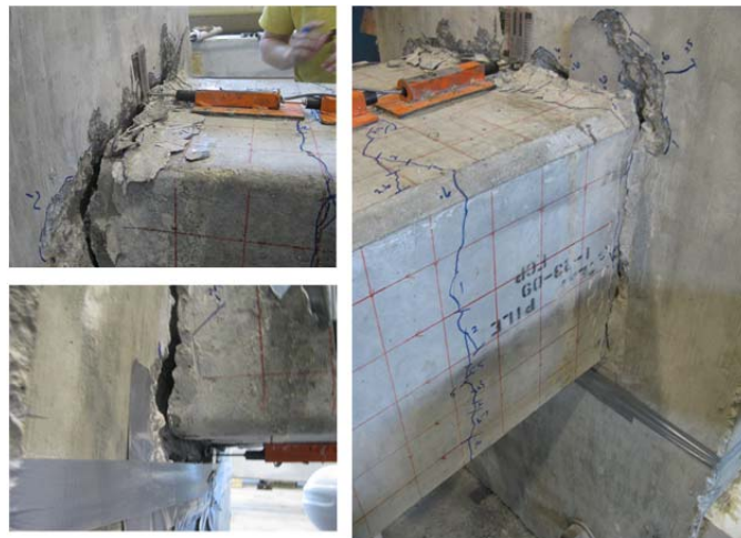
Figure 6.15 Damage Locations - Specimen IB-18-2
