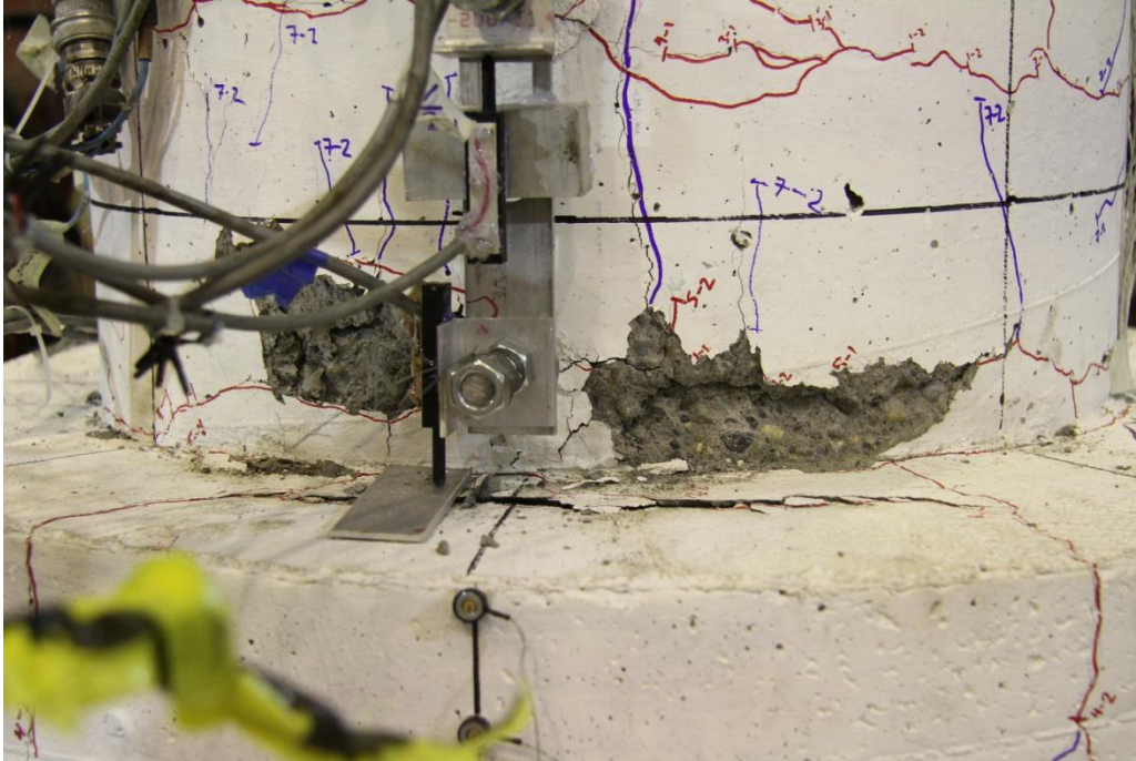
Figure C-0-2. DS-1 – First significant spalling occurred in the column in Cycle 7-2 (3.00/-3.14 percent drift)
