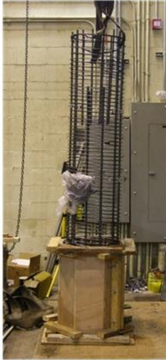
a). Column reinforcement
