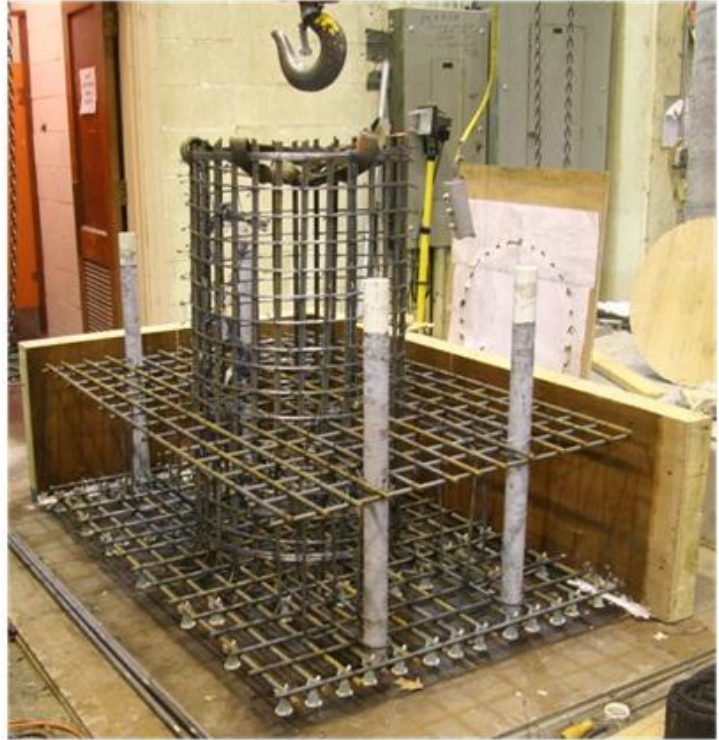
b). Shaft-Footing reinforcement
