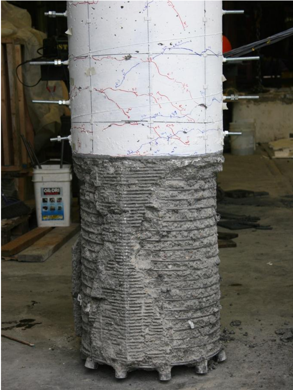
Figure C-0-13. DS-2 – Column damage after cyclic testing
