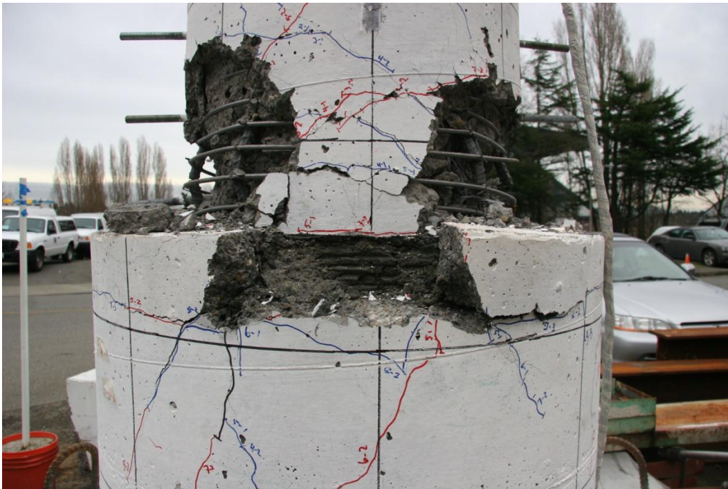
Figure C-0-6. DS-1 – Column damage after cyclic testing
