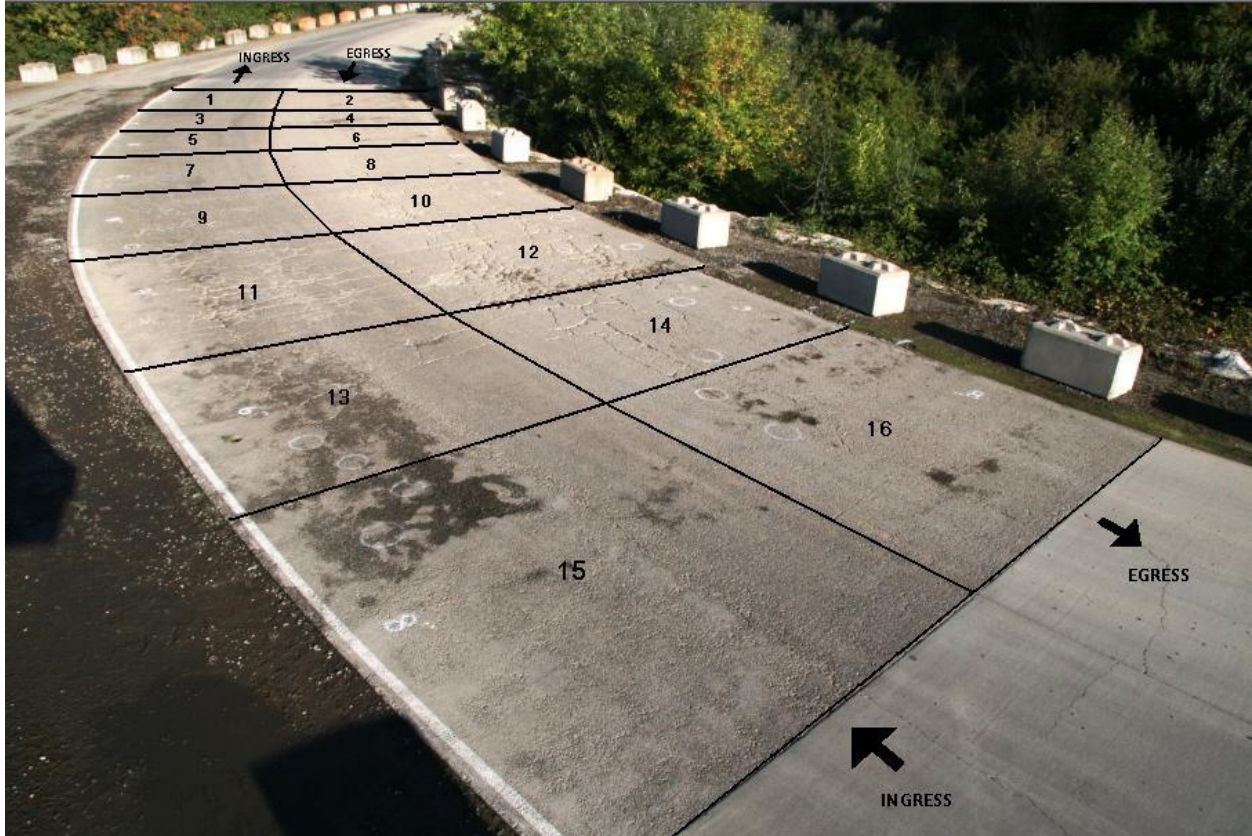
Figure 3.1: Photo of pervious concrete placement at Salem, OR (Goede, 2009)
