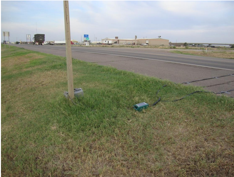
FIGURE 32 Pneumatic Road Tubes and Bluetooth Data Logger at Location “A”
