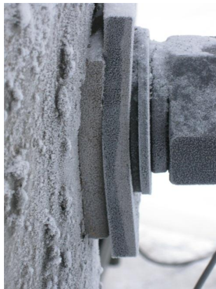
Figure 2.24: Bearing failure of test frame at reaction pile.
