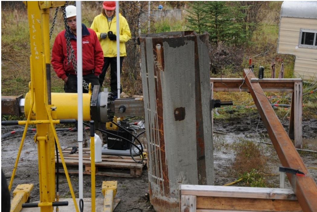
Figure 2.21: Reaction pile at final September load increment.
