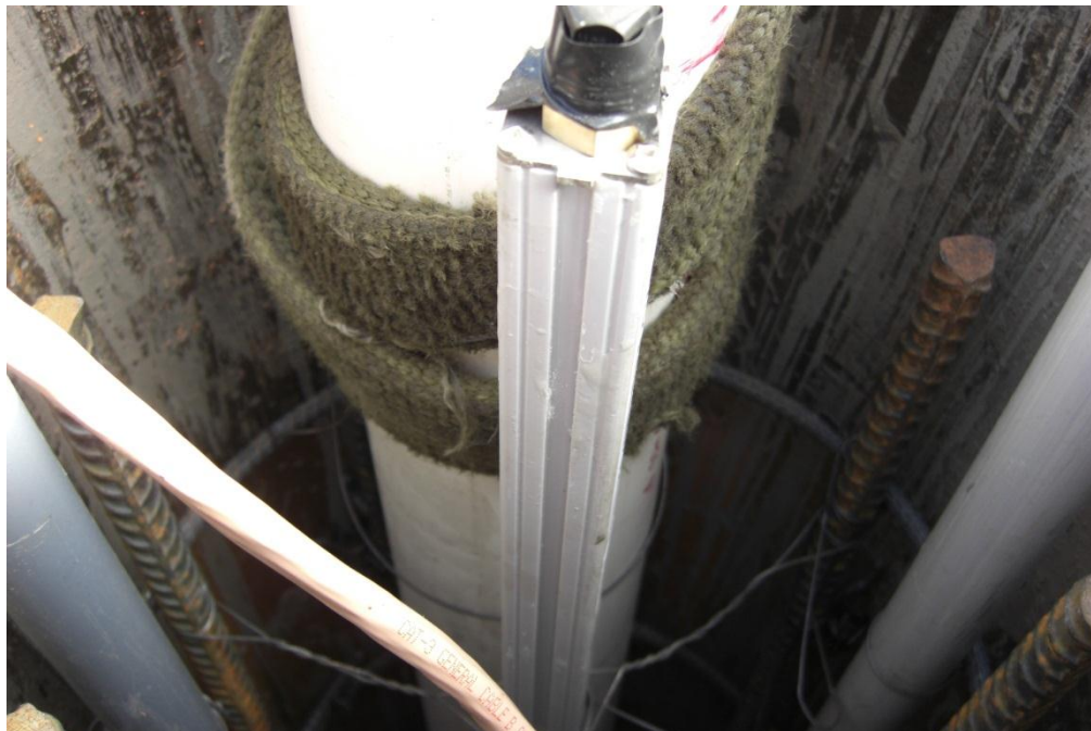
Figure 2.7: Inclinometer as installed in the test pile.
