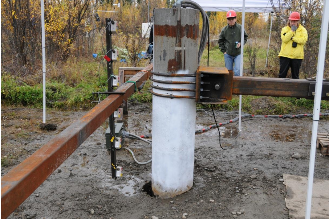
Figure 2.20: Test pile at final September load increment.
