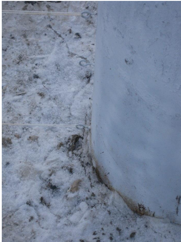
Figure 2.26: Soil crack at 150 kips, January test.
