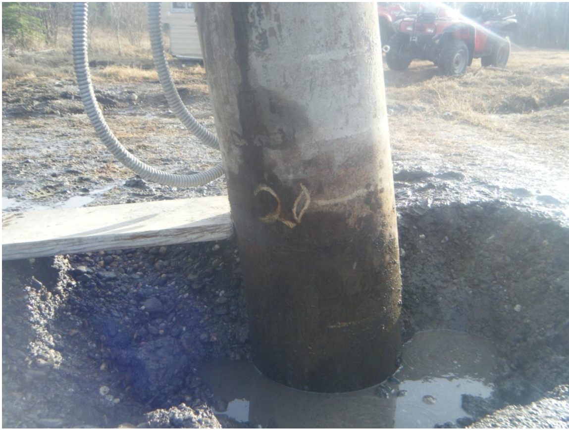
Figure 2.54: Excavation of south pile tested March 2010.
