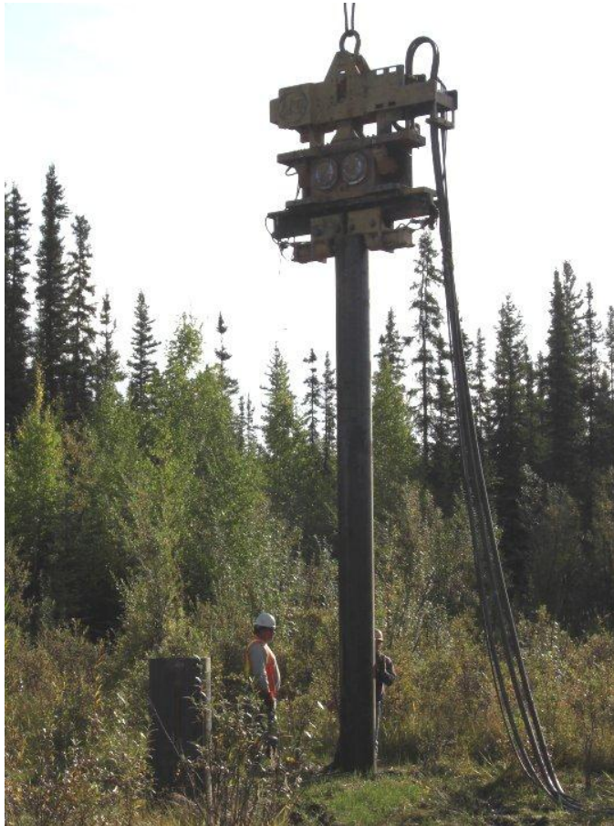
Figure 2.9: Installing a test pile using a vibration head (photo by INE staff).
