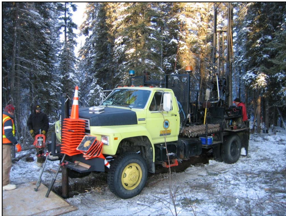
Figure 2.4. NRMS truck-mounted CME 45B drill centered over the trench at TH08-1650.
