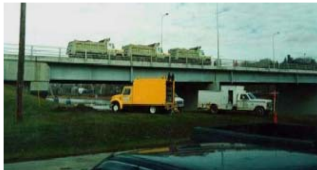
Fig. 21.25 Load testing of the Joffre Bridge with three loaded trucks
