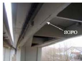
(c) Deformation measurement of a concrete bridge deck
