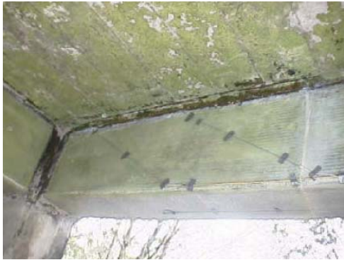
Fig. 13.2 Sensors mounted onto glass epoxy
