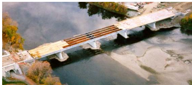
Fig. 21.23 The Joffre Bridge in Sherbrooke, Québec. During reconstruction in 1997
