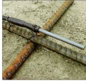
Fig. 18.7 Probe mounted just above Rebar
