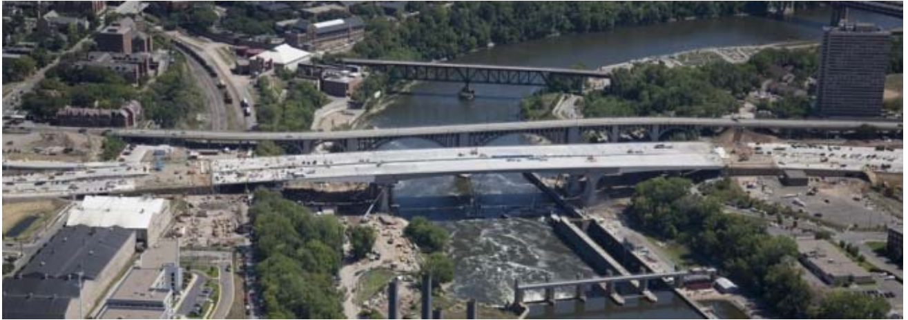
Fig. 21.1 The new I-35 Bridge
