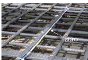
(b) Embedded in concrete
