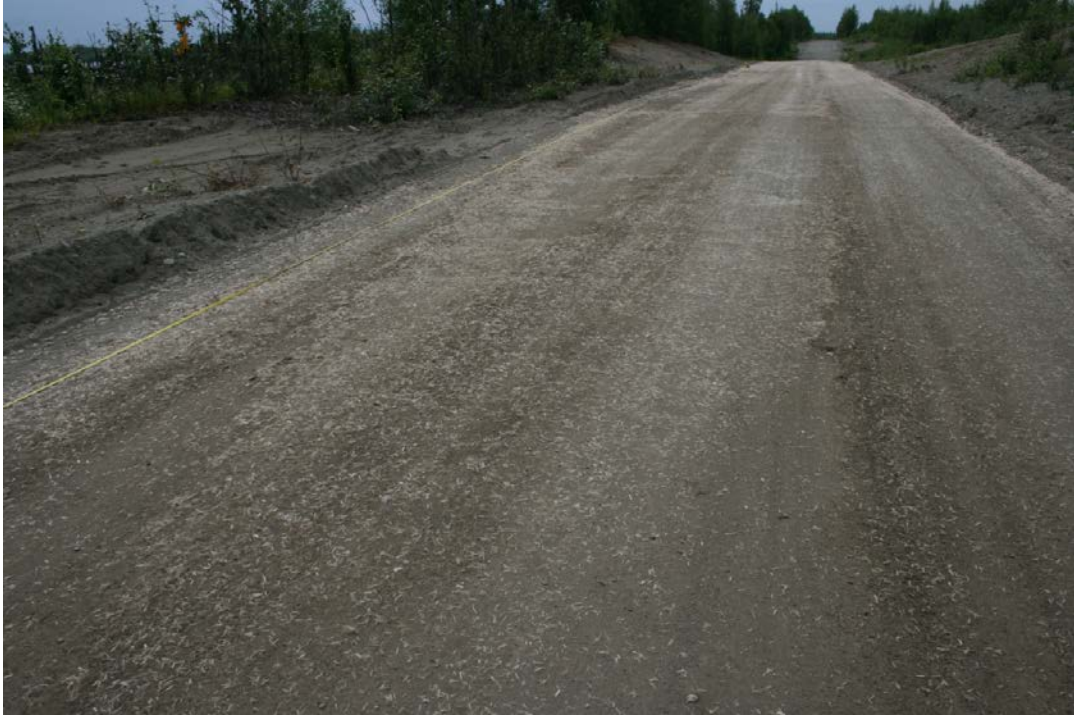
Figure 18: Roadway one week after construction
