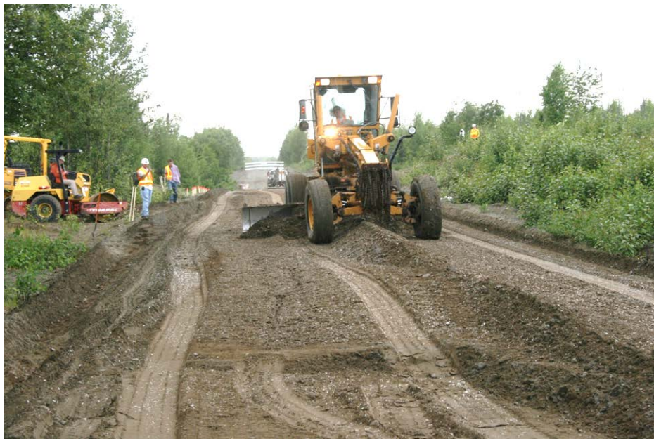
Figure 15: Shaping and grading
