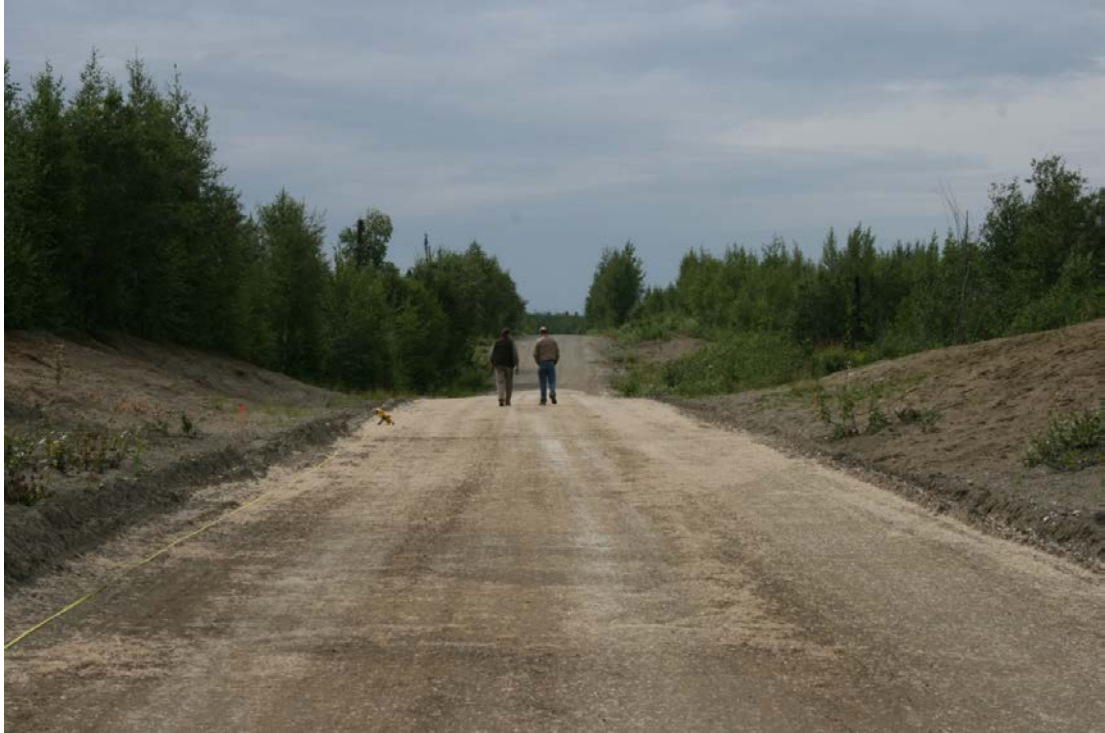
Figure 19: Roadway three weeks after construction (August 28 th , 2010)
