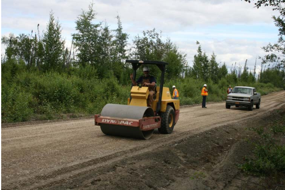
Figure 16: Compacting roadway
