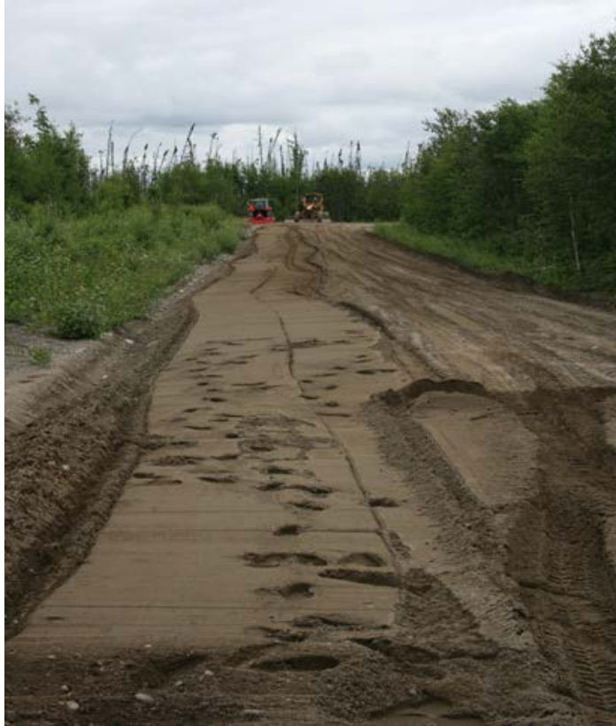
Figure 11: Roadway after being "fluffed"
