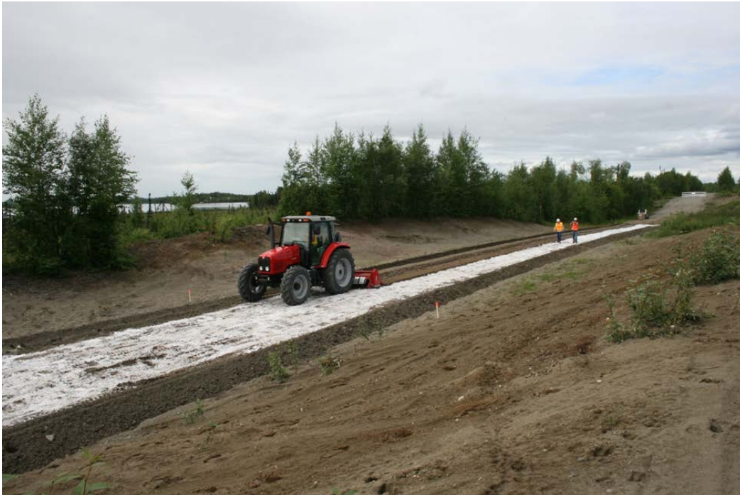
Figure 12: Achieving uniform application of fibers
