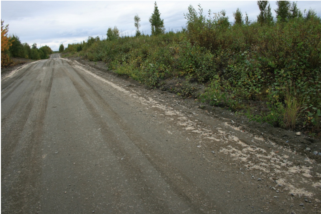
Figure 20: Test section September 7, 2010
