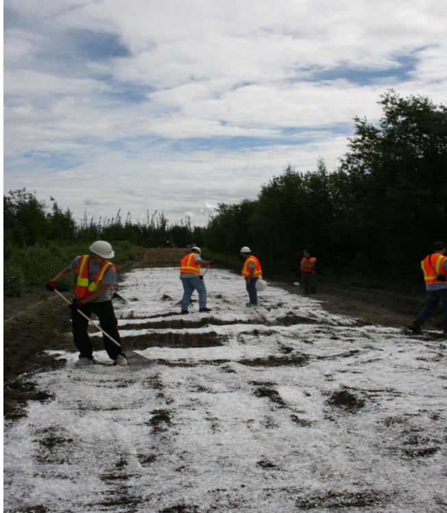
Figure 12: Achieving uniform application of fibers
