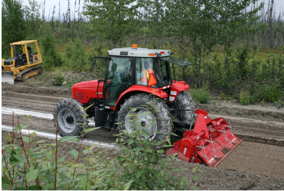
Figure 14: Final mixing of Soil-Sement and geofibers
