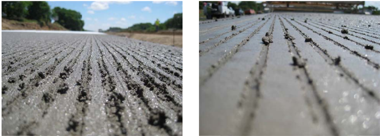
Figure 10. Photographs of newly constructed and textured PCCP surfaces.
