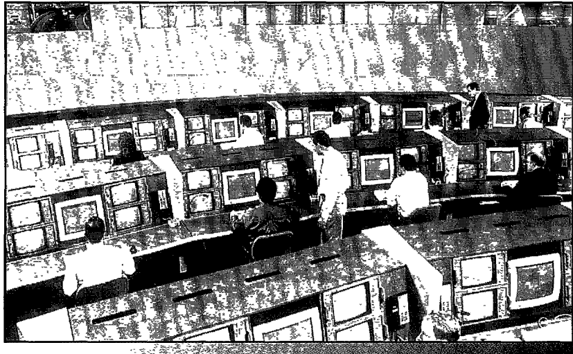
TransGuide Control Center, San Antonio
