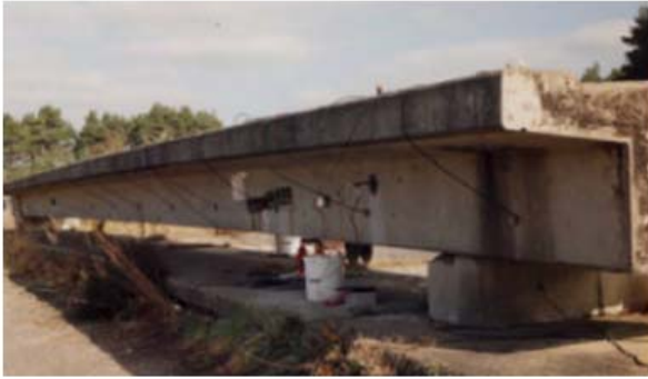
Instrumented Bank Lane Unit
